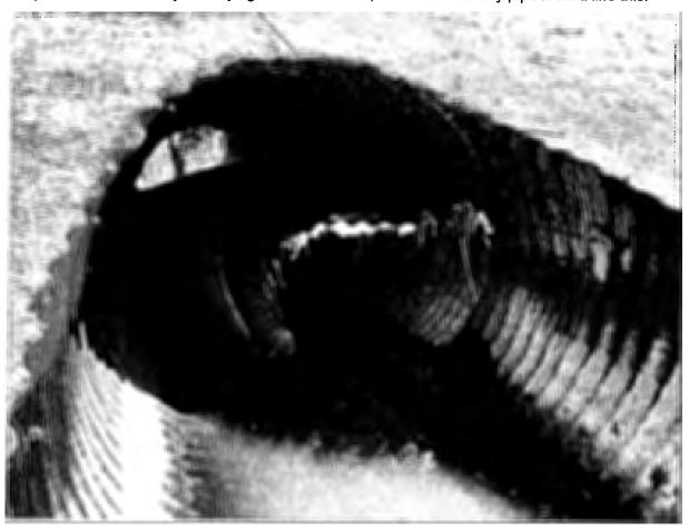
Our bridge technologist examined this culvert and noted that much of the granular backfill had washed out around this pipe, leaving about 20 feet of unsupported concrete deck. The crossing was immediately closed to all traffic.
