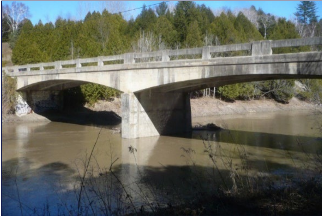
Bridge No. 9 West Elevation View
