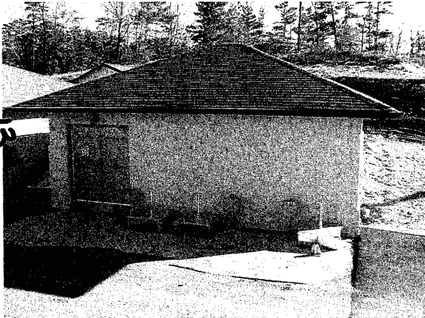
1. SBR WWTP - Stouffville, ON
