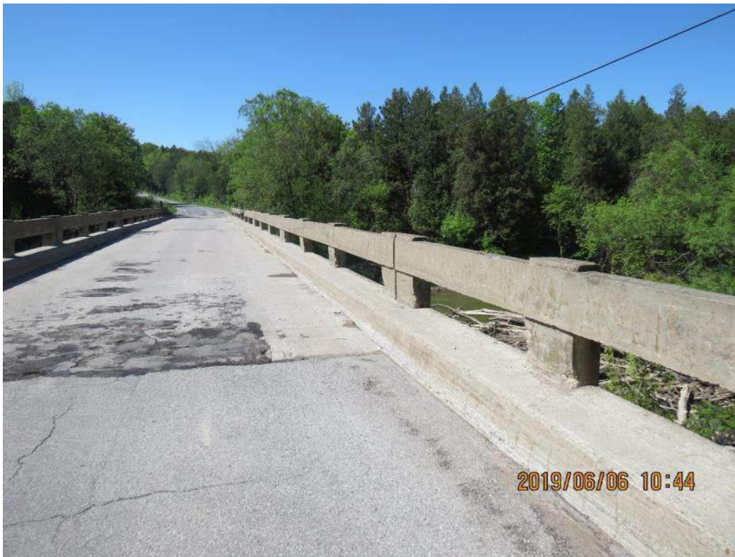
IMG_1394 Typical West Curb (2 of 2)
