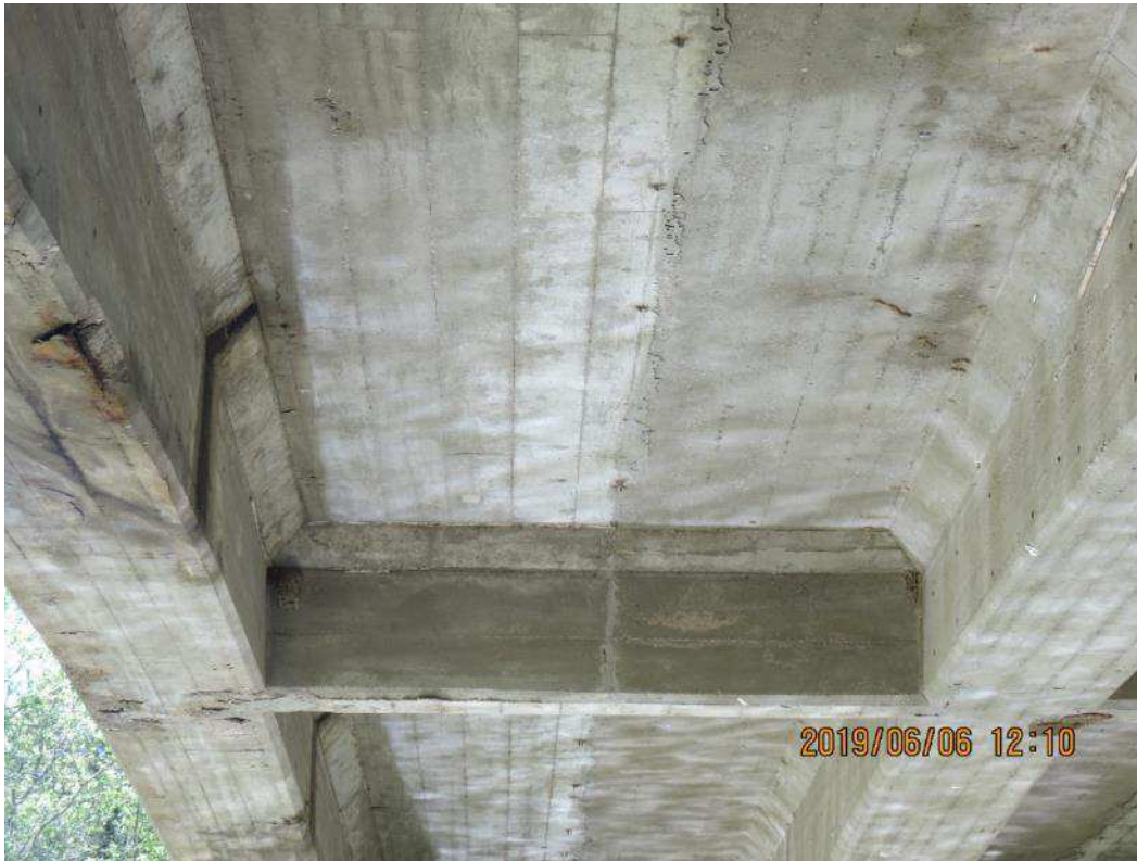
IMG_1786 Typical North Diaphragm
