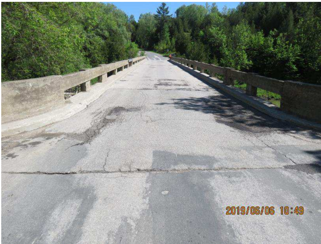
IMG_1431 South Approach and Deck Joints
