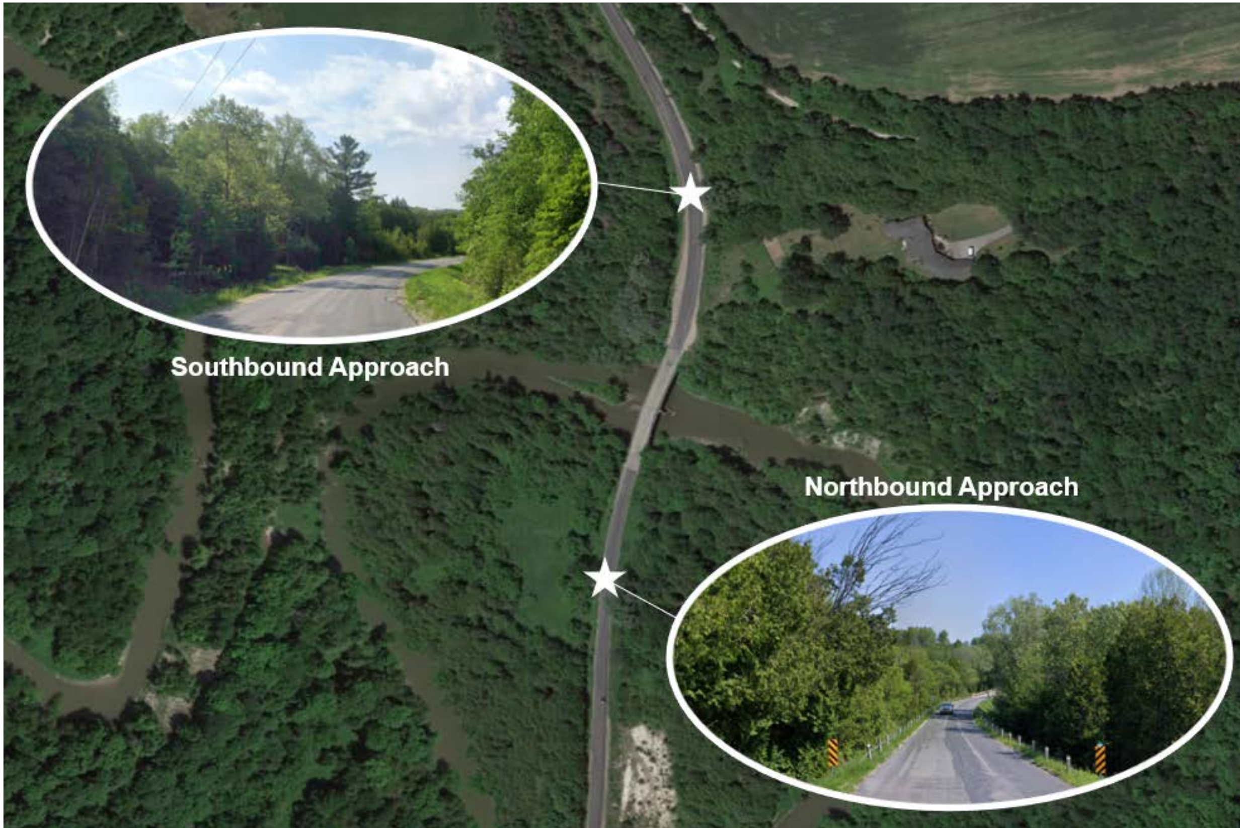
Figure 6: 5 th Line Approaches to Bridge No. 9
