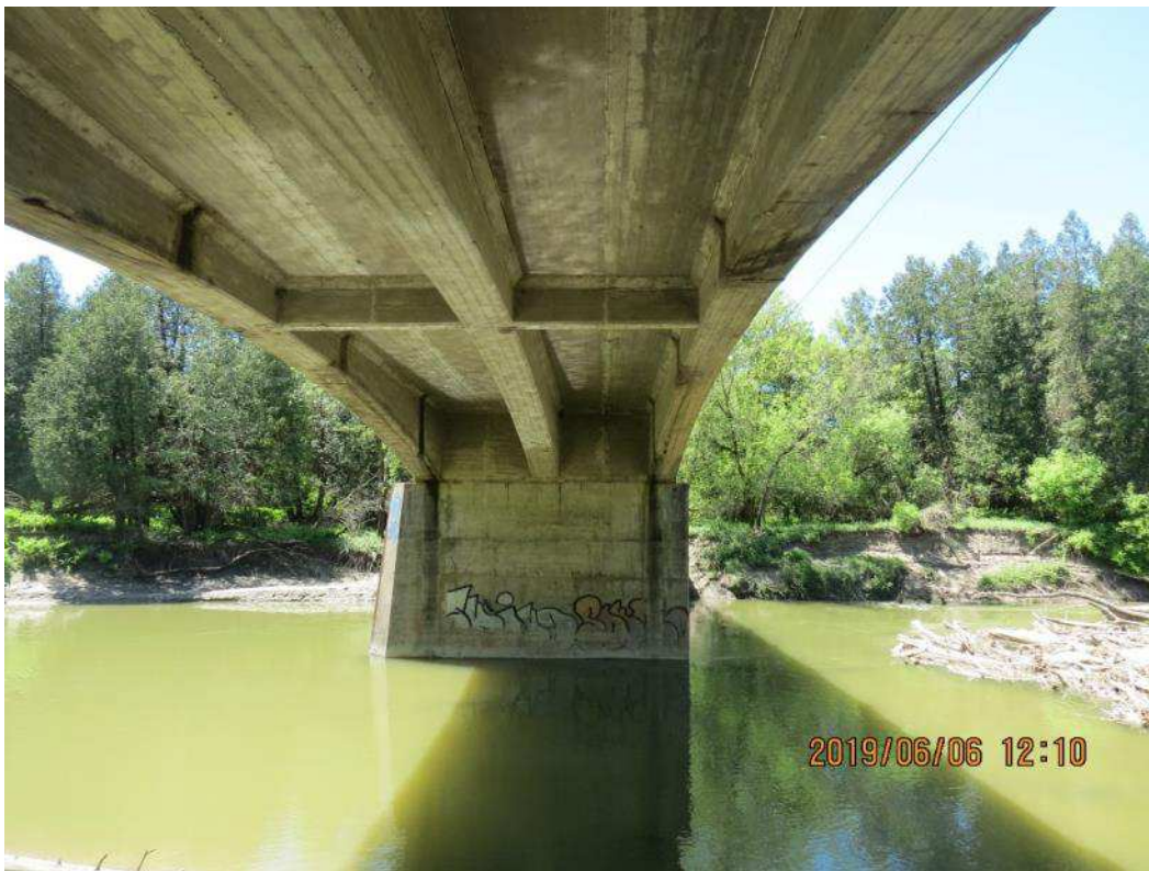
IMG_1789 North Span Soffit (Looking South)
