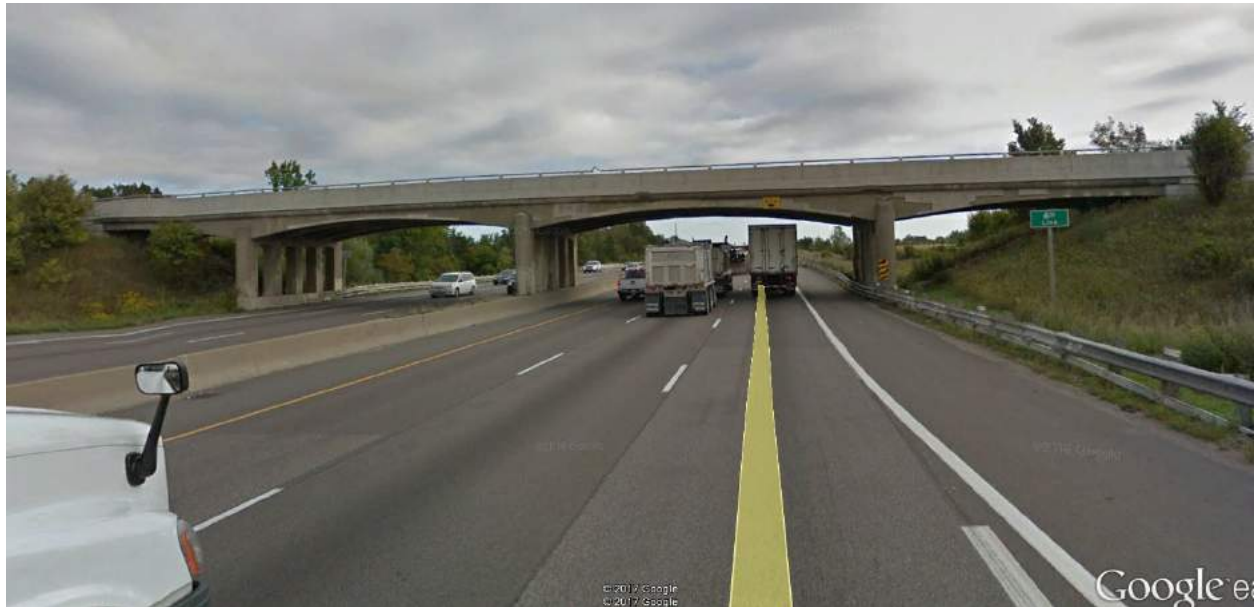
Figure 10: Highway 401-Sixth Line Underpass, a four-span T-beam structure constructed in 1958 (Google Streetview)
