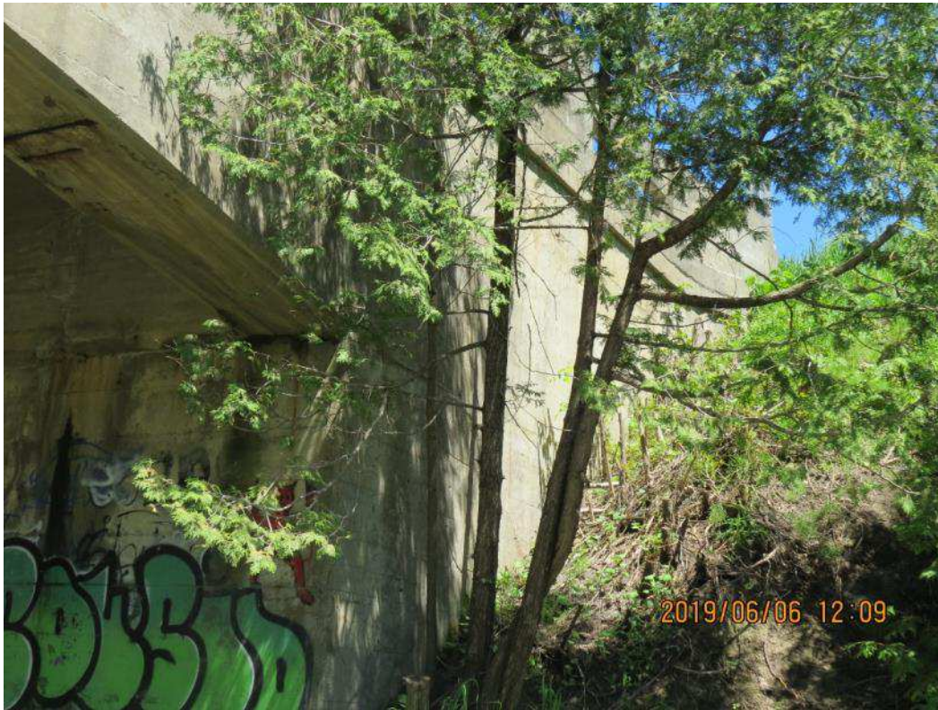
IMG_1776 Northeast Wingwall (2 of 2)
