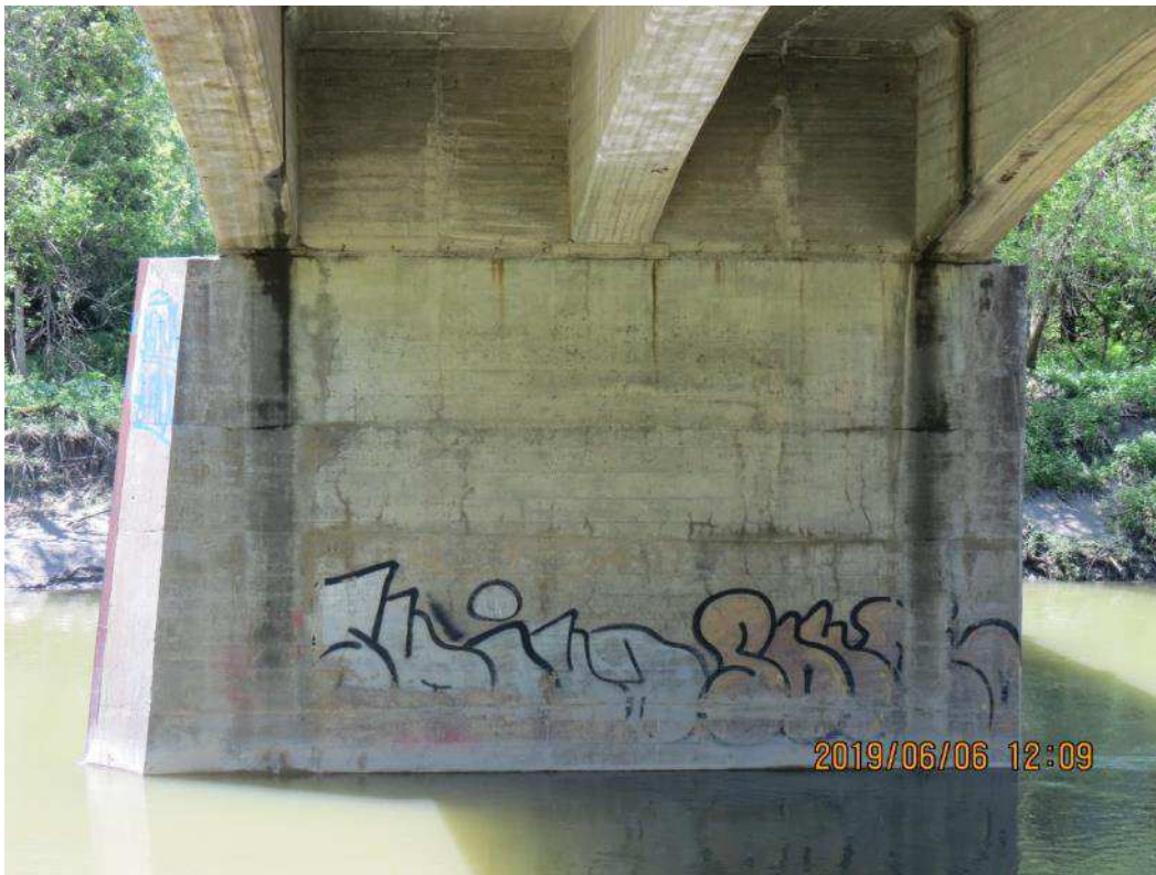
IMG_1782 Center Pier North Face
