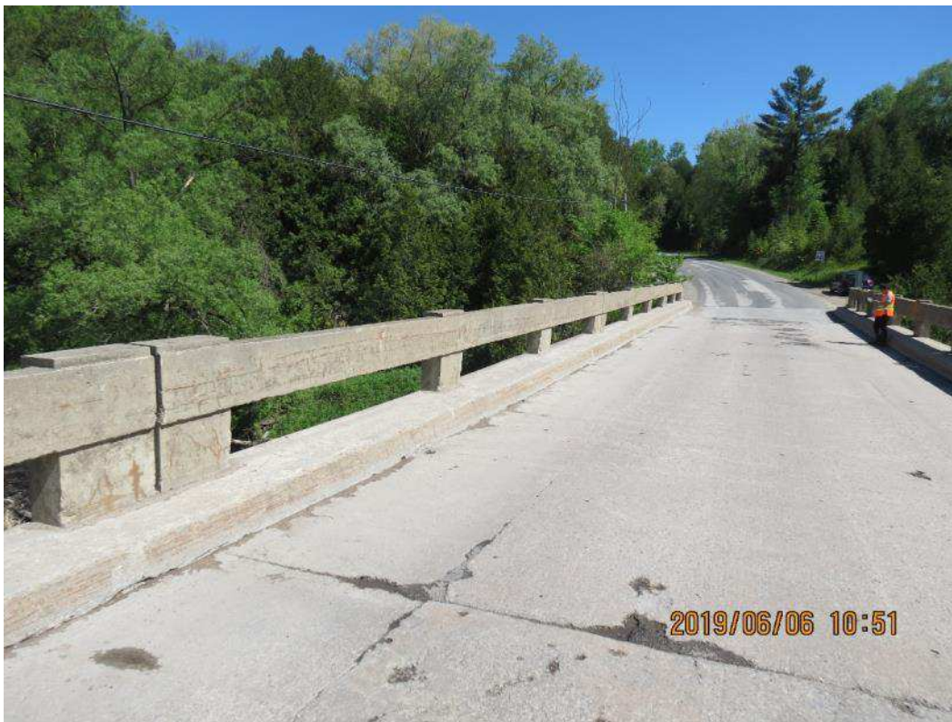
IMG_1446 Typical West Post Inside Face
