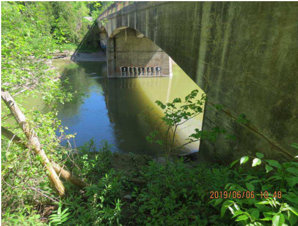
IMG_1426 Northwest Embankment (1 of 2)
