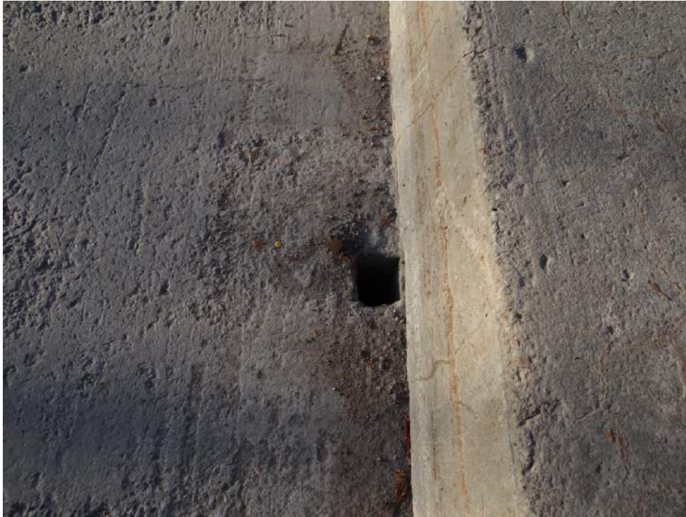
Plate 16: Drainage hole through the bridge deck, with the curb at right.
