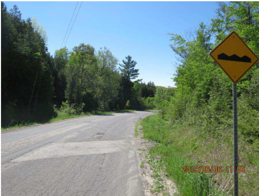
IMG_1555 Road North of Bridge (2 of 3)
