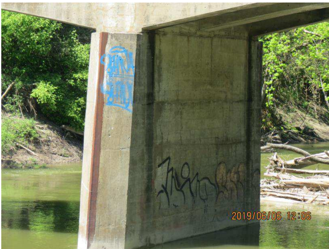
IMG_1764 Center Pier East Side (1 of 2)
