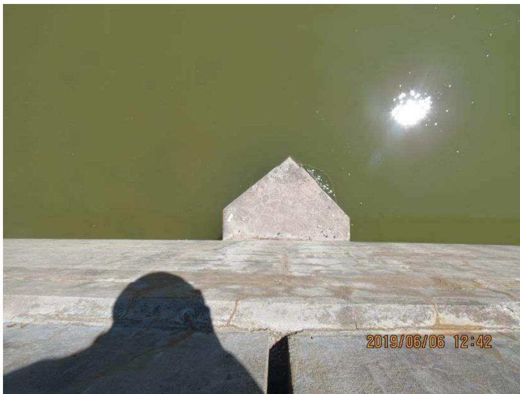
IMG_1861 Center Pier East Side (2 of 2)
