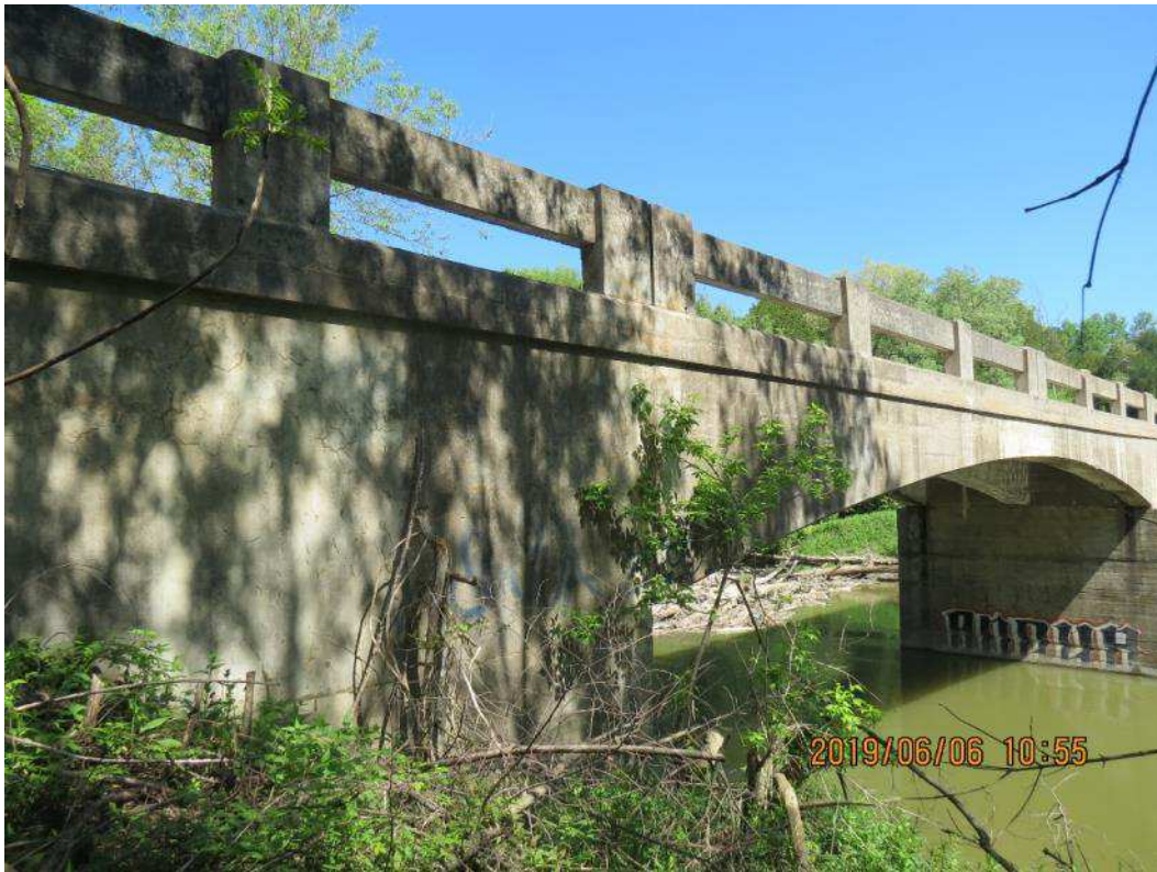
IMG_1485 Southeast Wingwall
