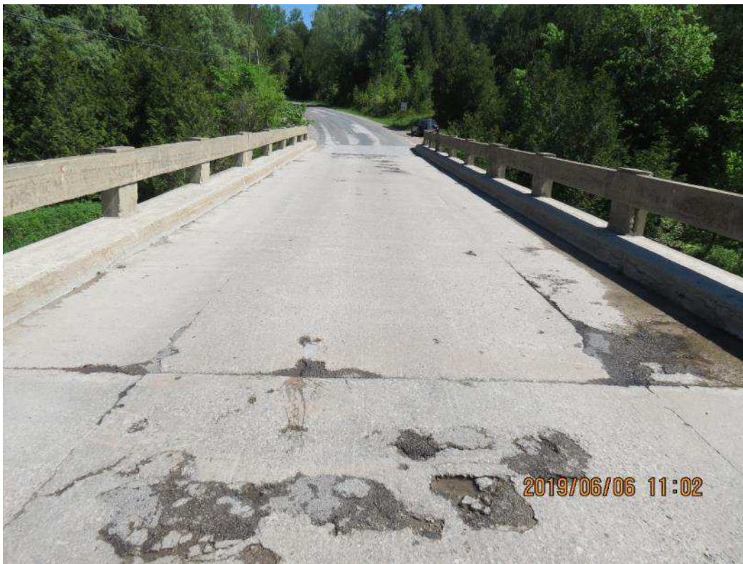
IMG_1533 Center Span Deck Joint
