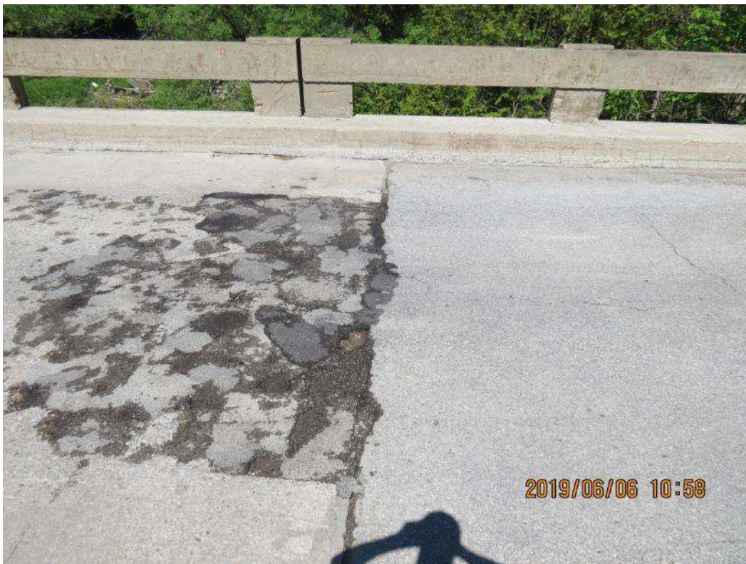
IMG_1509 North Joint at Deck (2 of 2)
