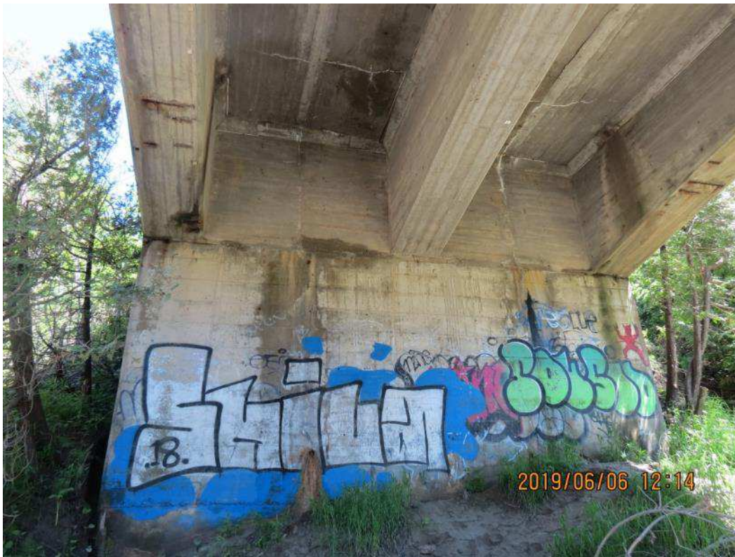
IMG_1817 North Abutment Wall
