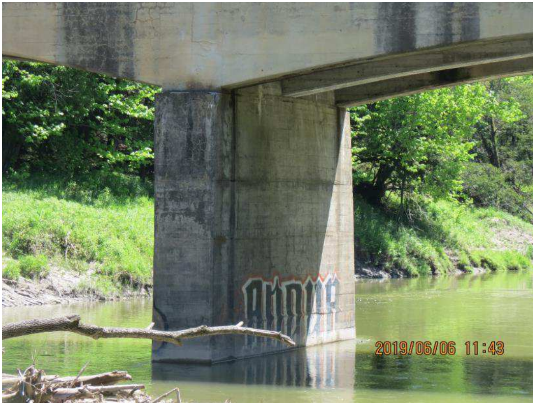
IMG_1659 Center Pier West Side (1 of 2)
