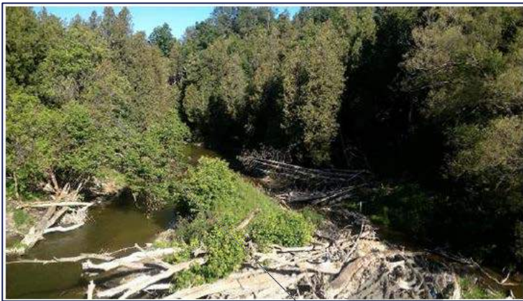
Downstream of Bridge, June 2021 Riverstone Environmental
