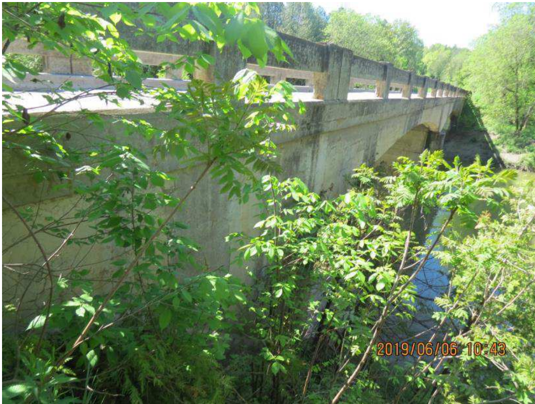
IMG_1388 Northwest Wingwall (1 of 2)
