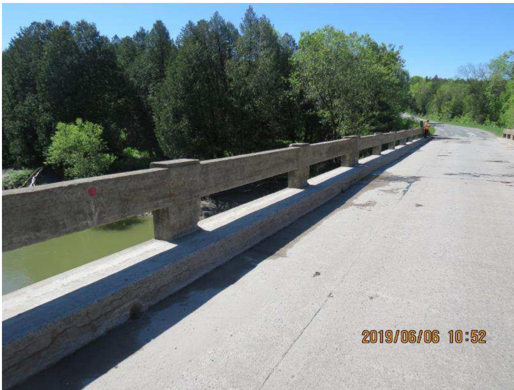
IMG_1462 Typical East Concrete Post Inside Face
