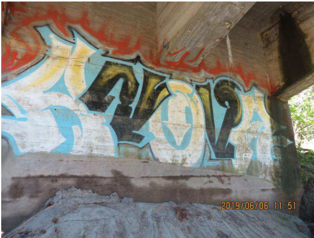
IMG_1710 South Abutment Wall
