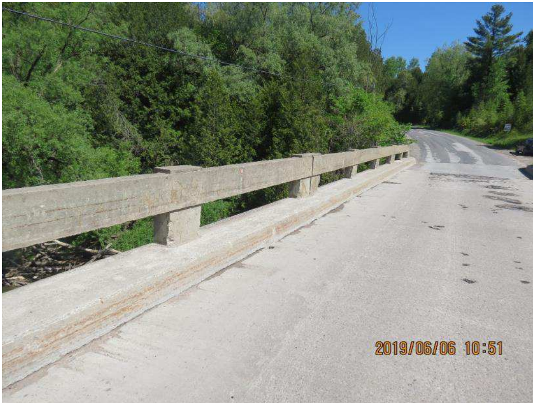
IMG_1447 Typical West Curb (1 of 2)
