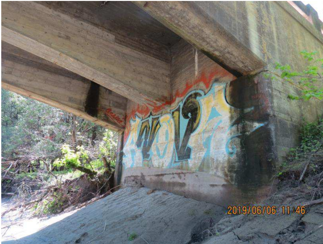
IMG_1666 South Girders (2 of 2)
