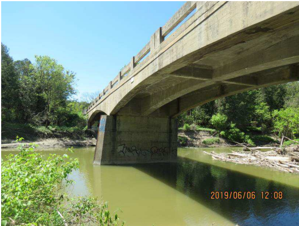
IMG_1768 Southeast Embankment (1 of 2)
