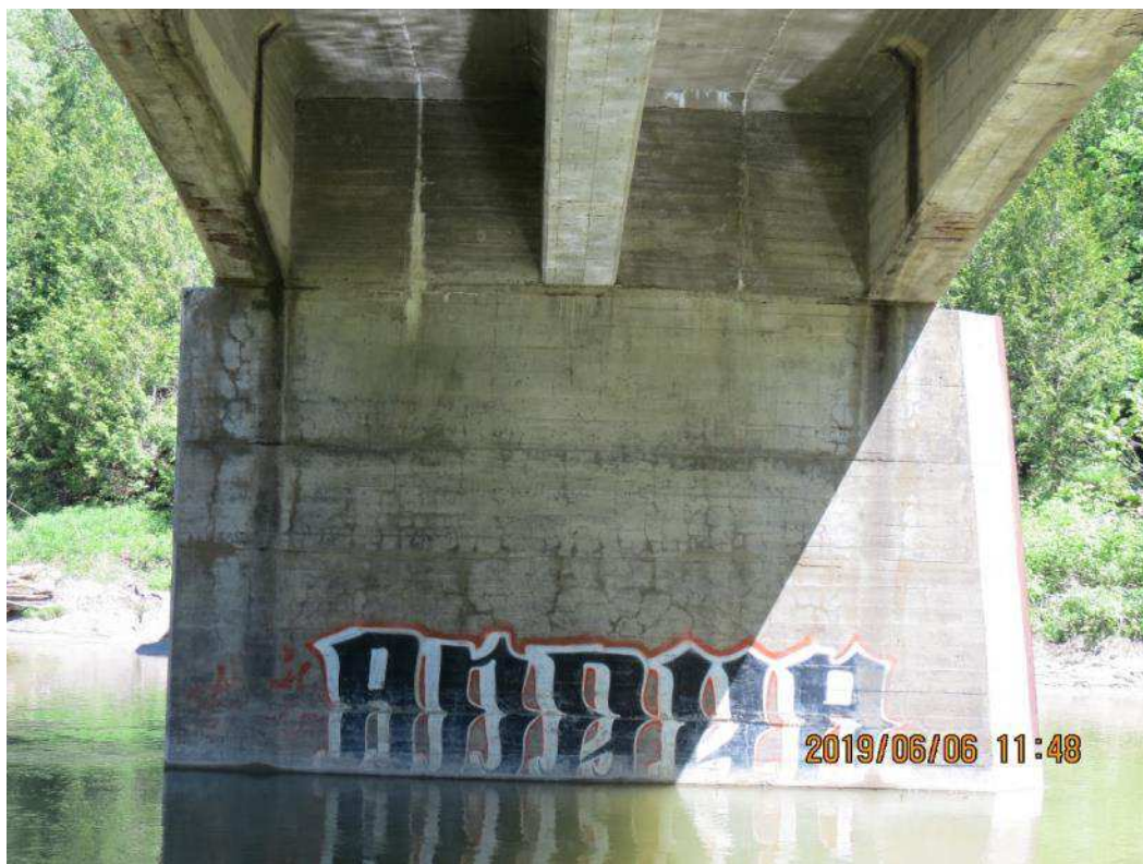
IMG_1686 Center Pier South Face
