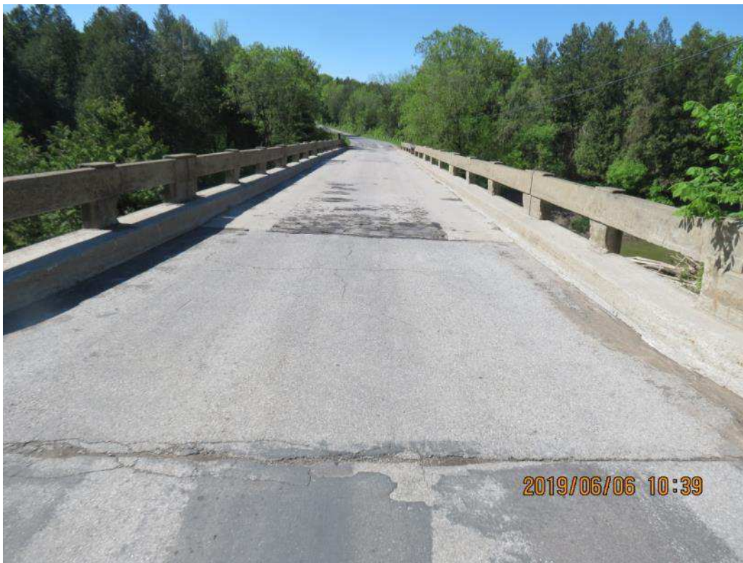
IMG_1361 North Approach & Deck Joints
