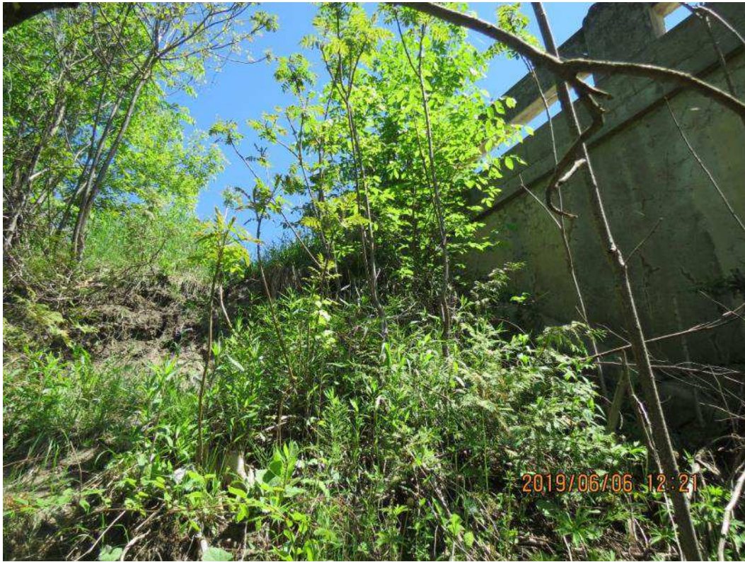
IMG_1856 Northwest Embankment (2 of 2)
