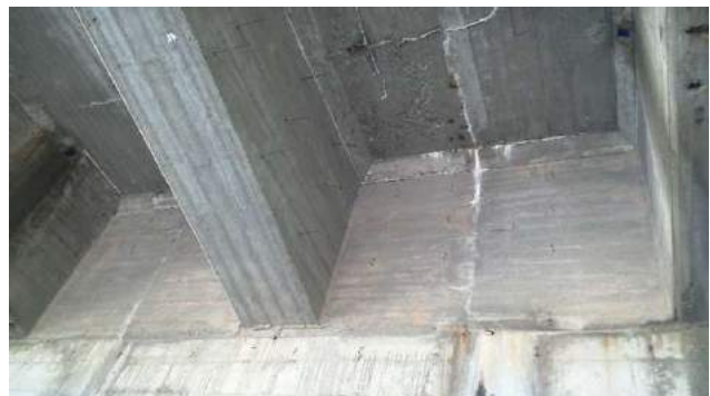
Photo 6. Facing north; underside of bridge (June 17, 2021).
