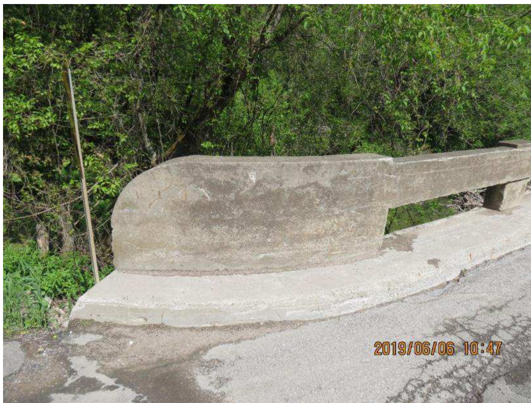
IMG_1418 West Railing South End Panel
