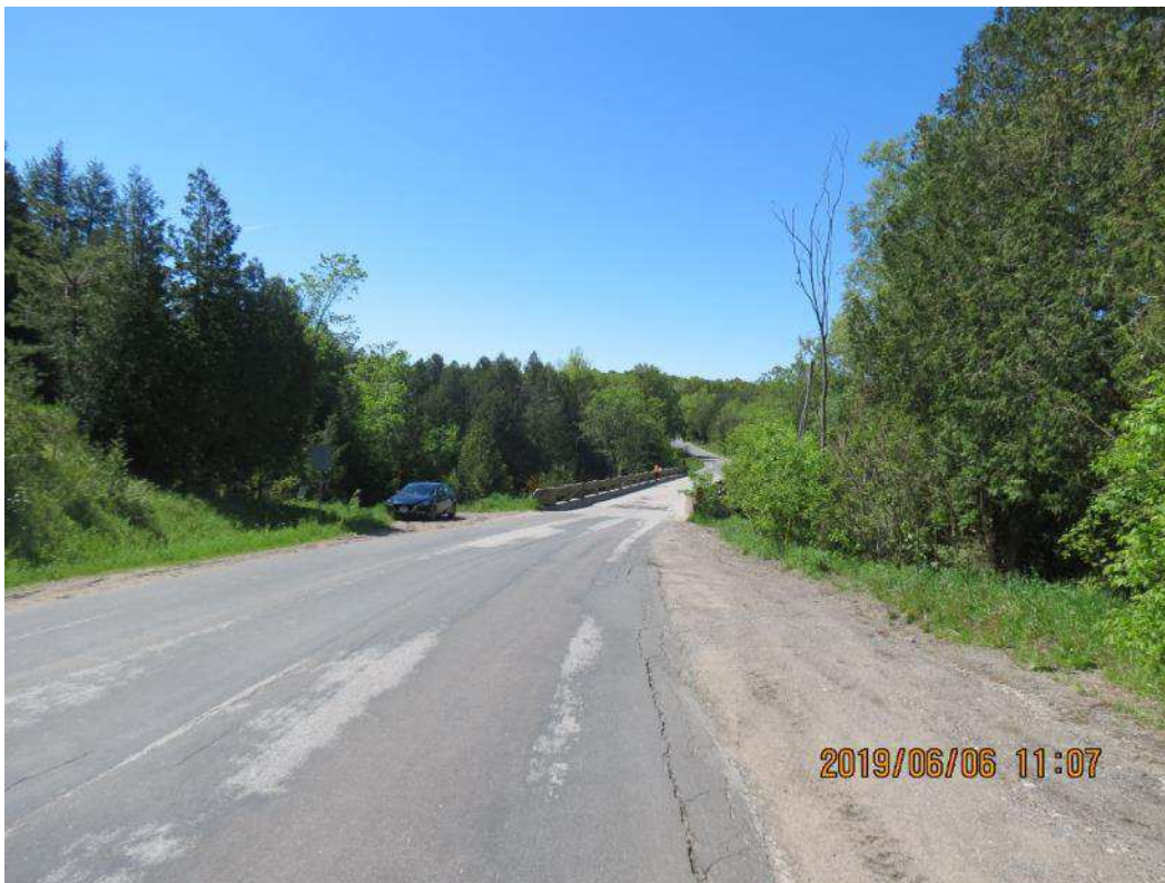
IMG_1559 Road North of Bridge (3 of 3)
