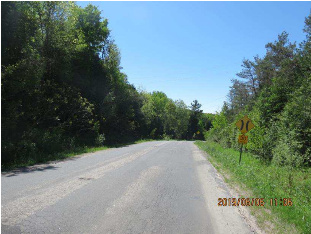
IMG_1551 Road North of Bridge (1 of 3)
