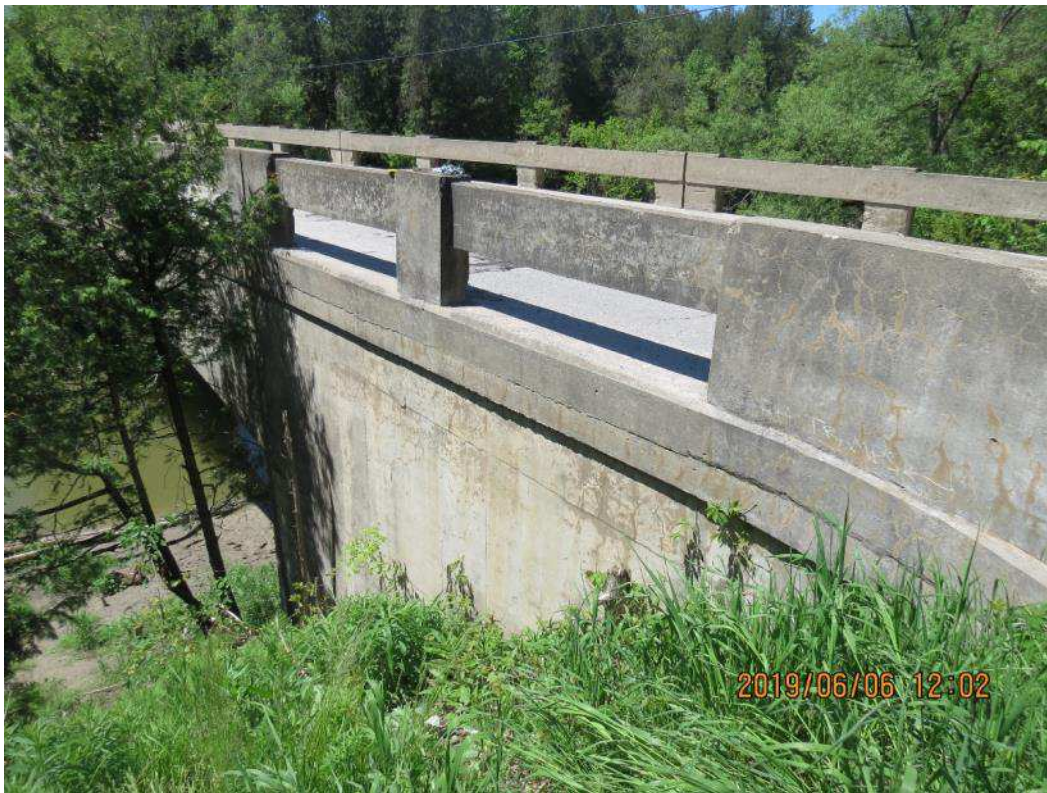
IMG_1743 Northeast Wingwall (1 of 2)
