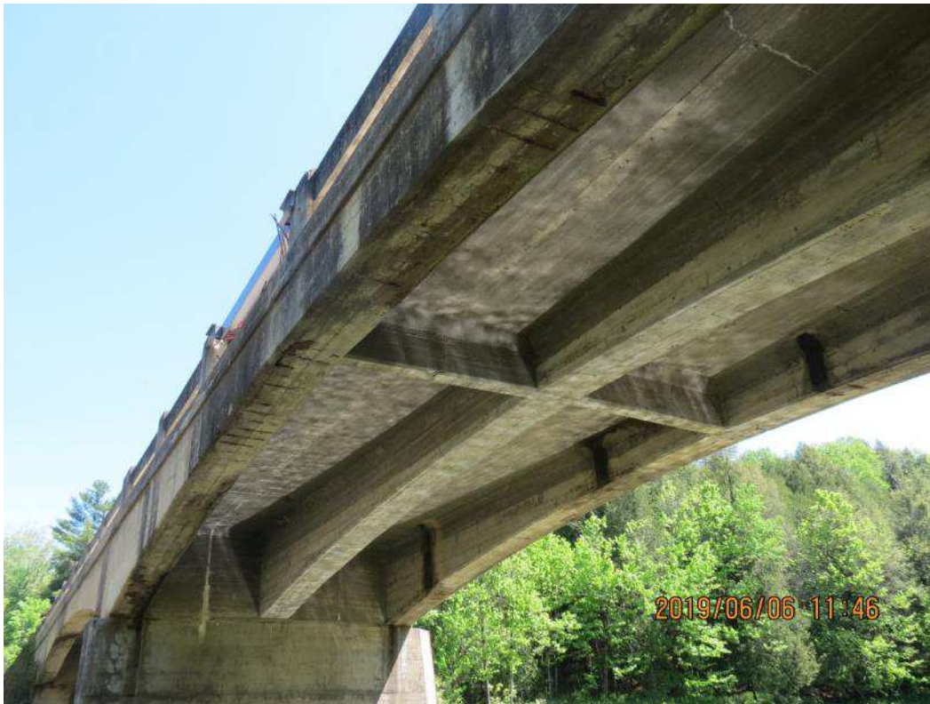
IMG_1670 South Girders (1 of 2)
