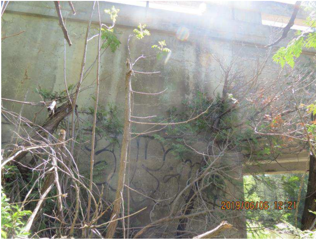
IMG_1854 Northwest Wingwall (2 of 2)
