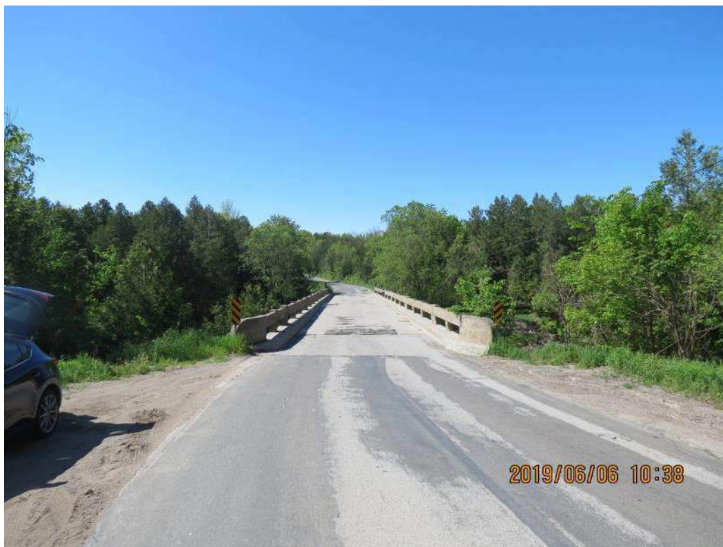
IMG_1357 Road over Structure Looking South
