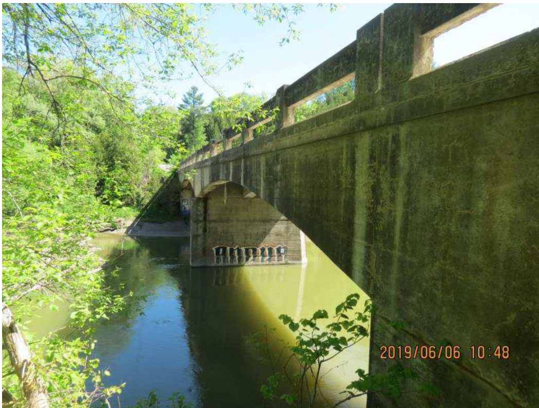
IMG_1427 West Fascia from South End
