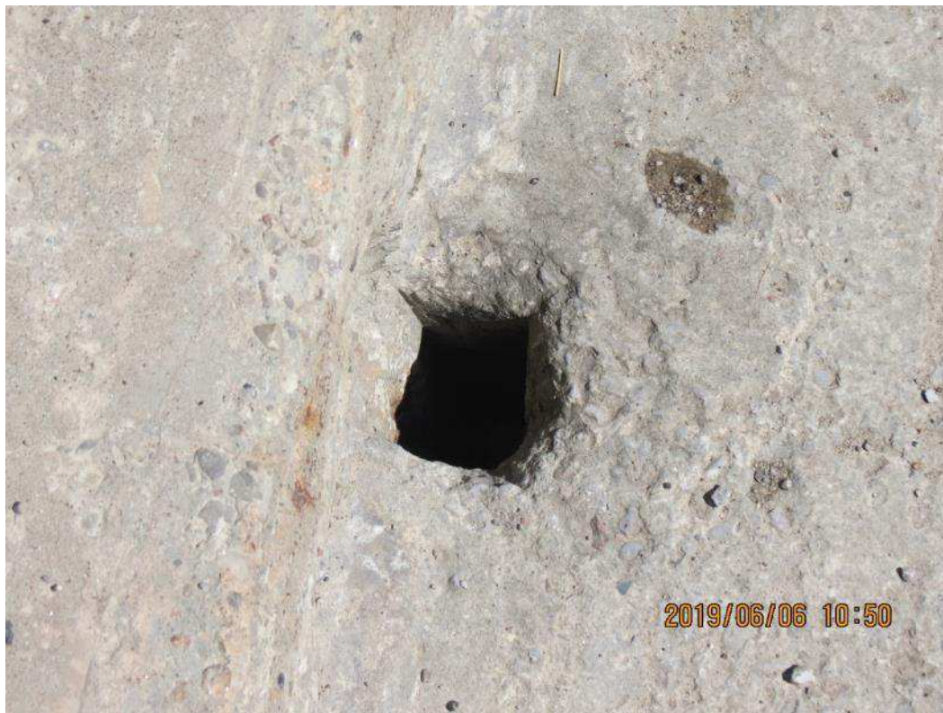
IMG_1442 Typical Deck Drain from Top of Deck
