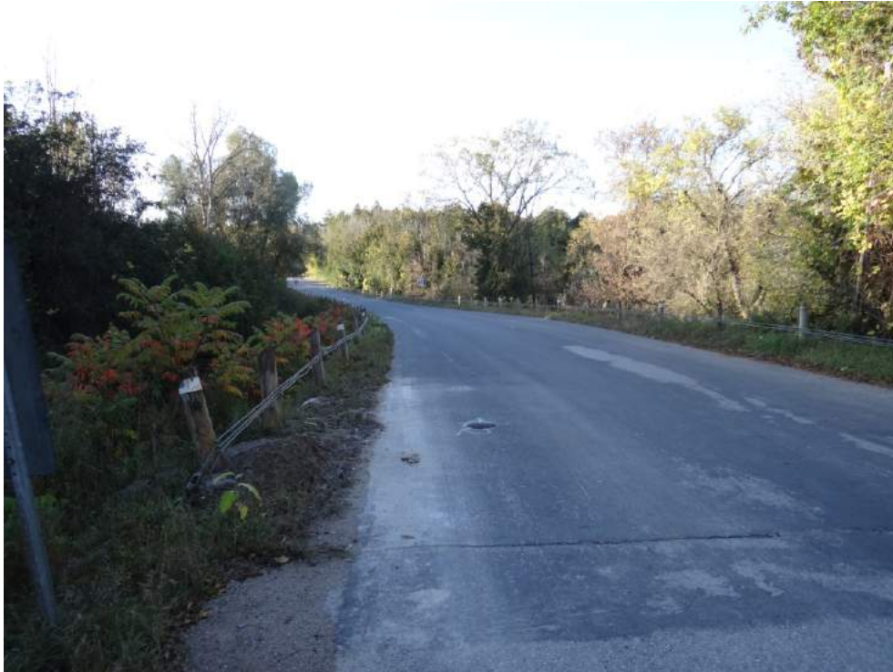
Plate 18: 5 th Line south of the subject bridge, looking south from the south approaches.
