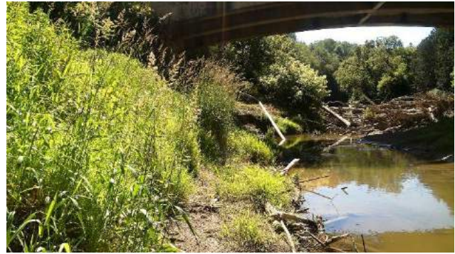
Photo 8. Facing east (upstream), under bridge along north bank; note log-jam along center of channel; approximate location of poorly-defined drainage feature outlet (June 17, 2021).
