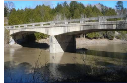
Bridge No. 9 West Elevation View (2019)
