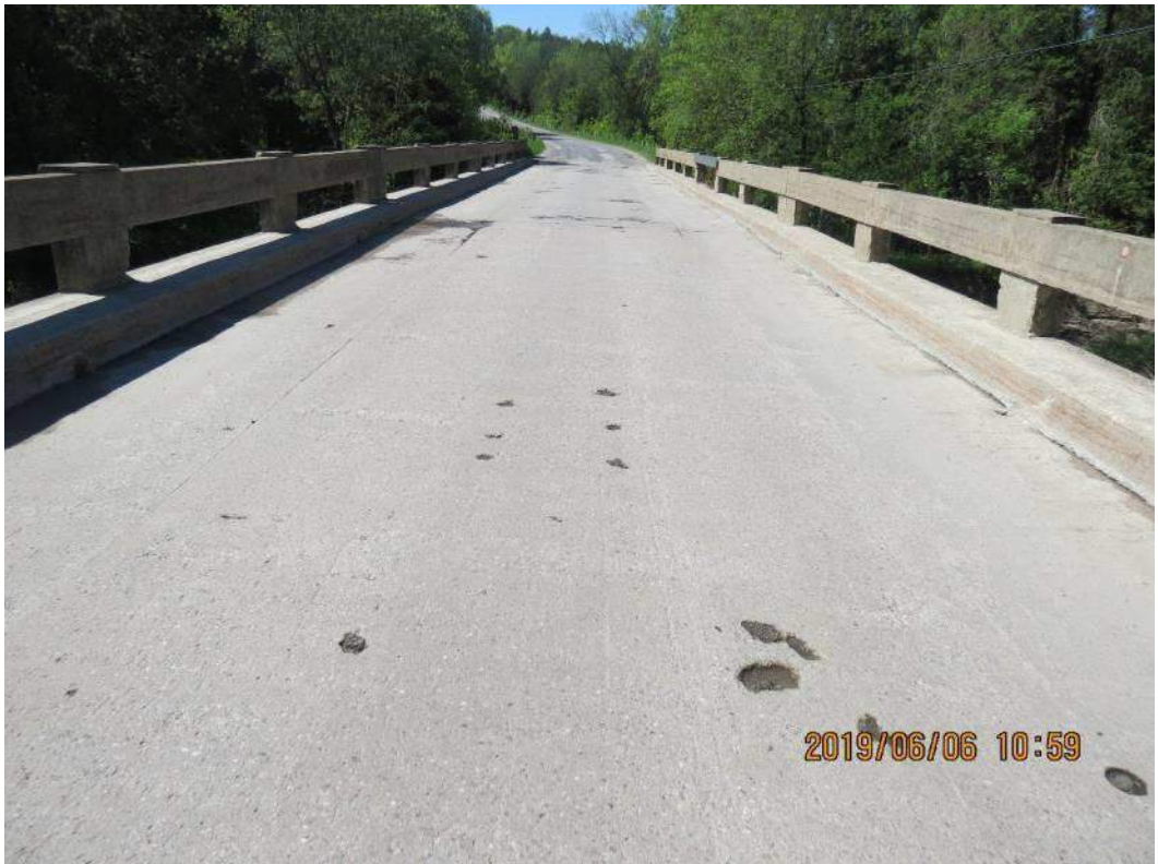
IMG_1512 Typical Deck Top
