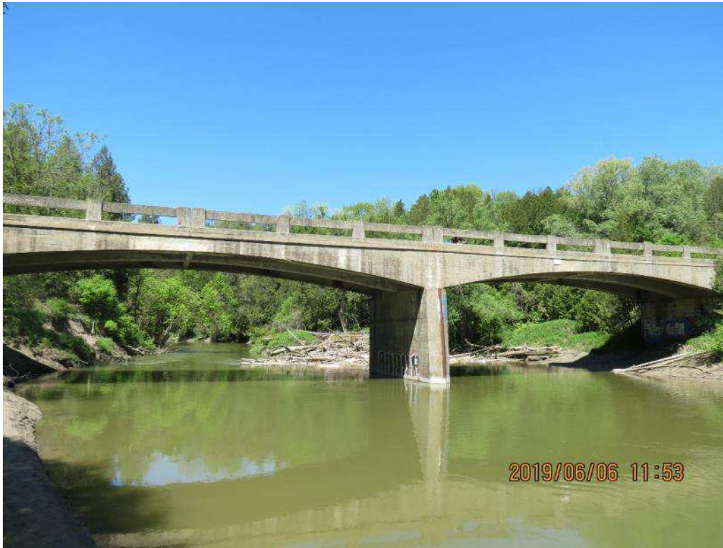
IMG_1726 East Elevation View
