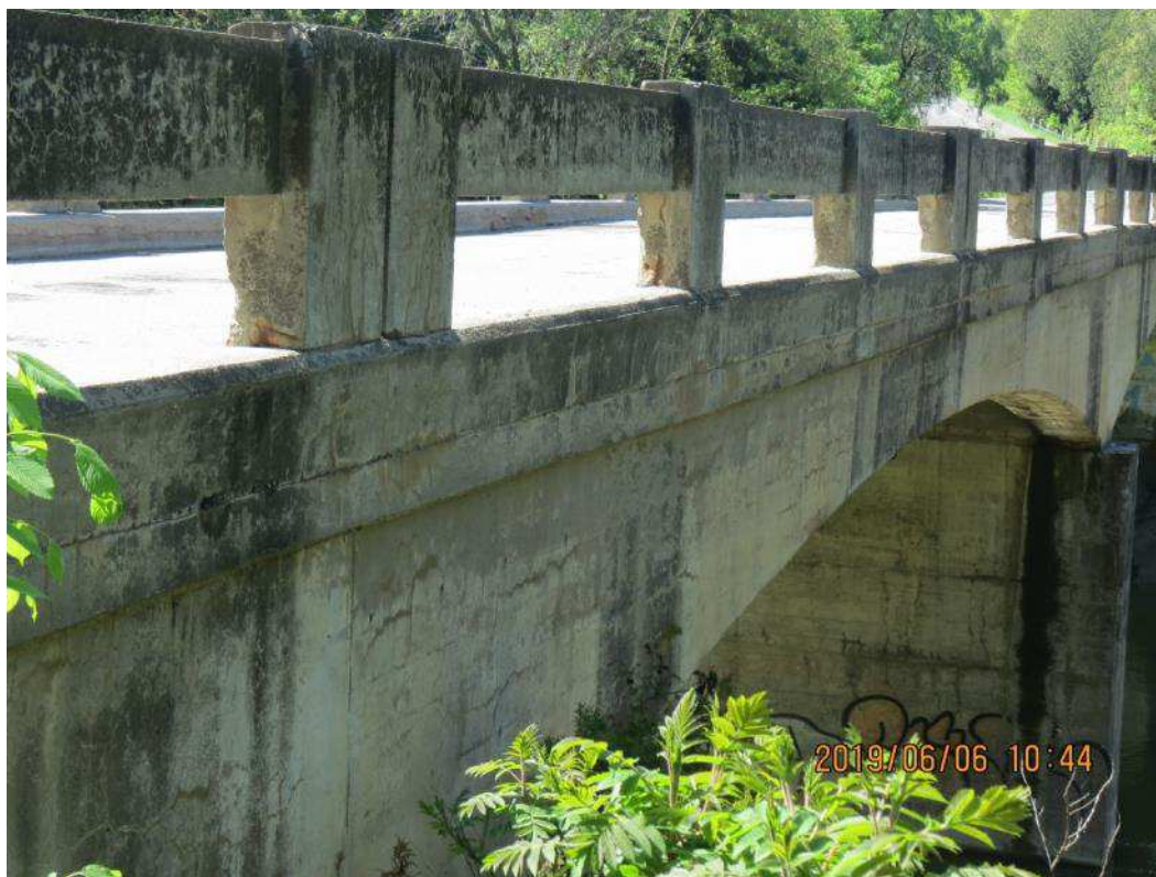
IMG_1390 West Railing Outside Face
