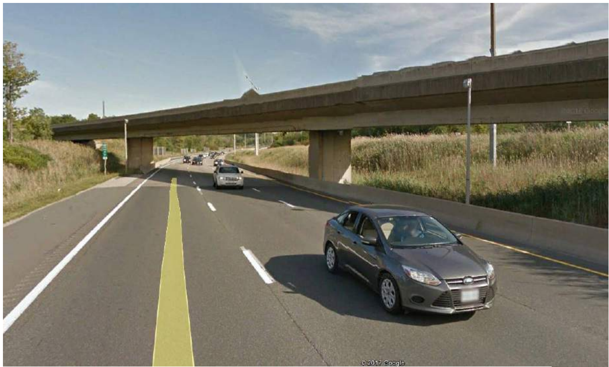
Figure 11: Highway 405-QEW Underpass, a three-span T-beam structure built in 1962 (Google Streetview)
