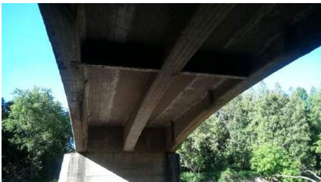
Photo 5. Facing south; underside of bridge (June 17, 2021).
