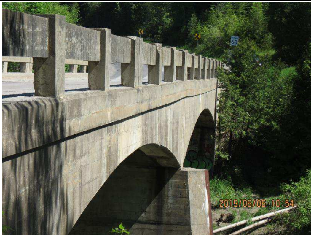
IMG_1481 East Railing Outside Face
