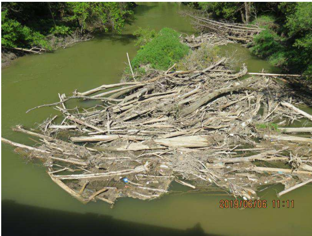
IMG_1572 Downstream Debris Buildup
