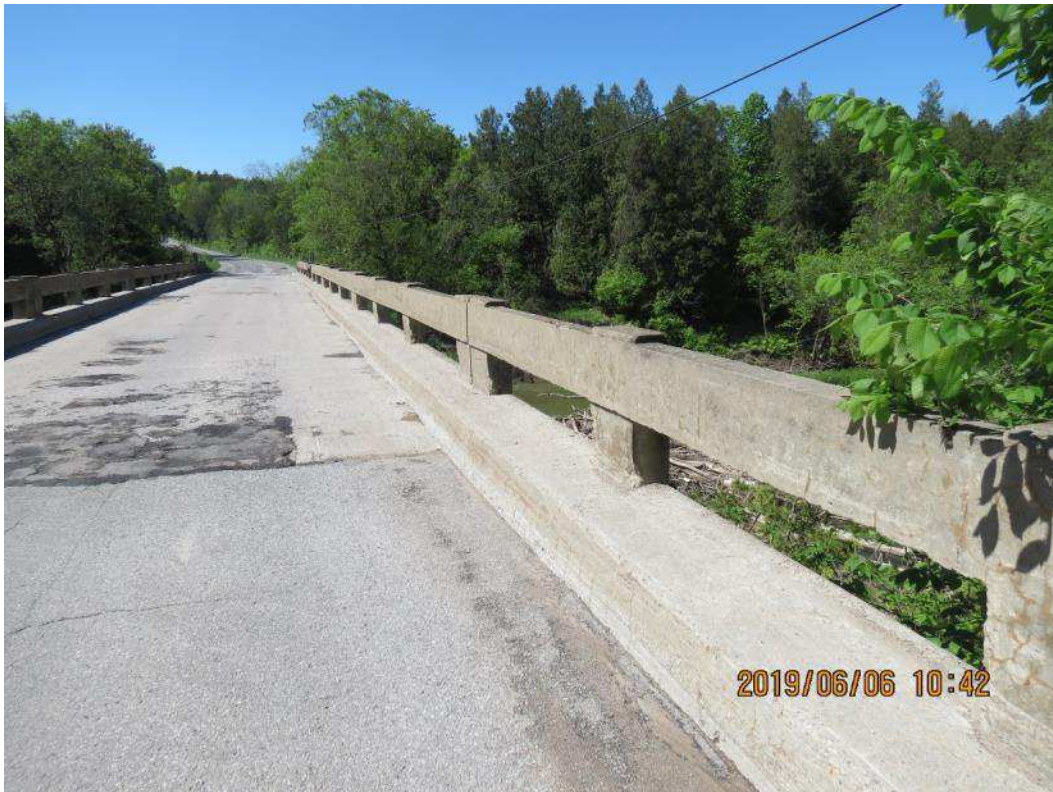
IMG_1379 West Railing Inside Face
