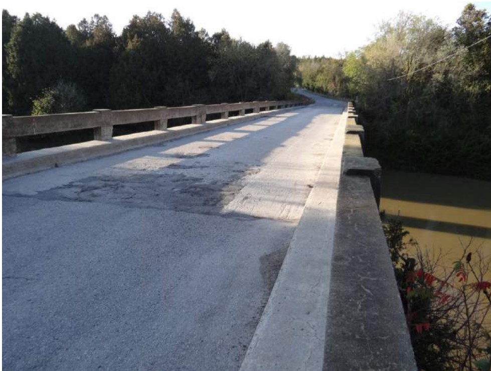
Plate 14: Bridge deck, looking south on 5 th Line over the structure.
