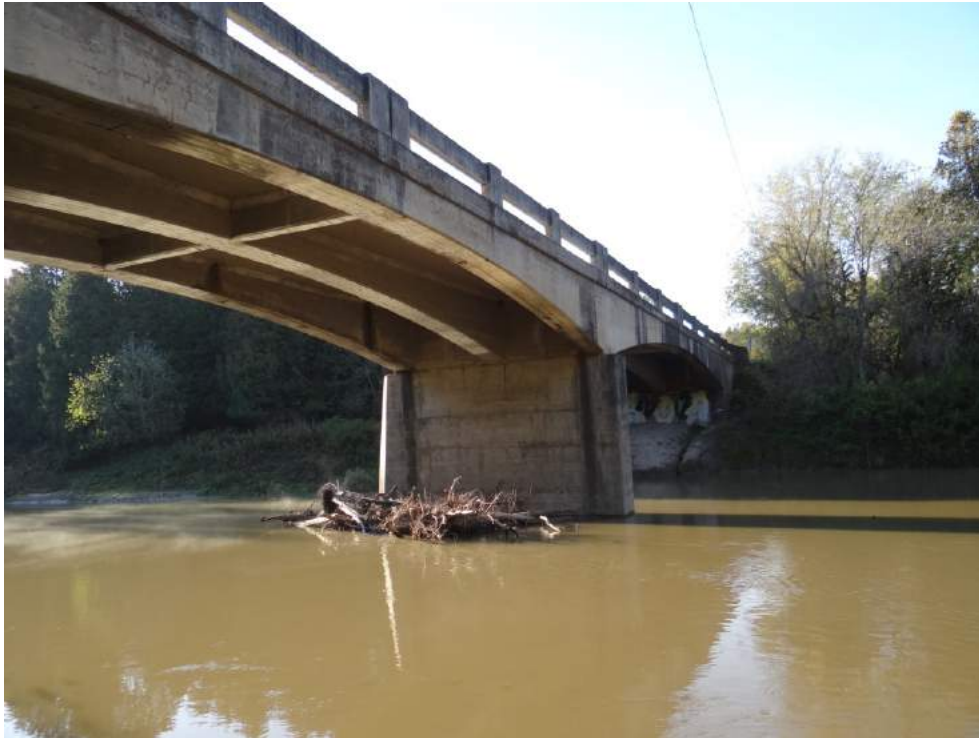
Plate 1: West elevation of the subject bridge, looking southeast.
