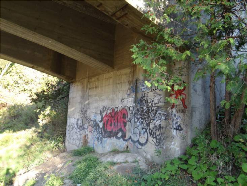
Plate 9: North abutment, looking northwest.
