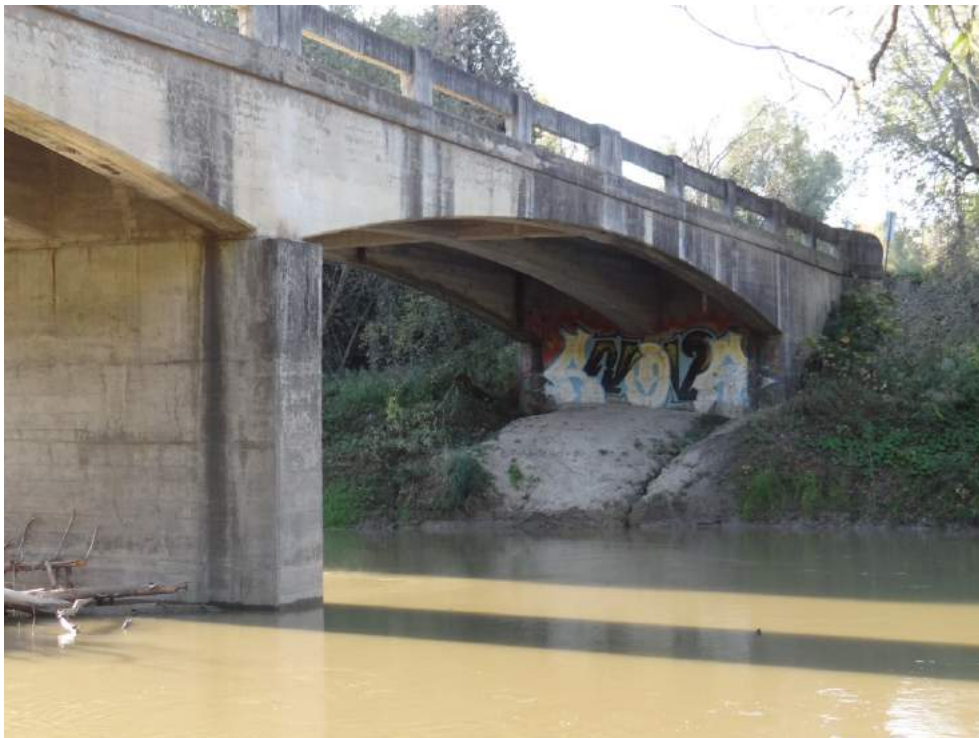
Plate 4: West elevation of the southern span and southern abutment, looking southeast.
