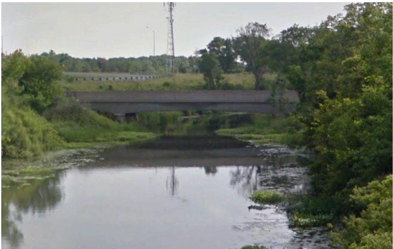
Figure 9: Lyon's Creek Bridge, a single-span T-beam structure built in 1941 (Google Streetview)
