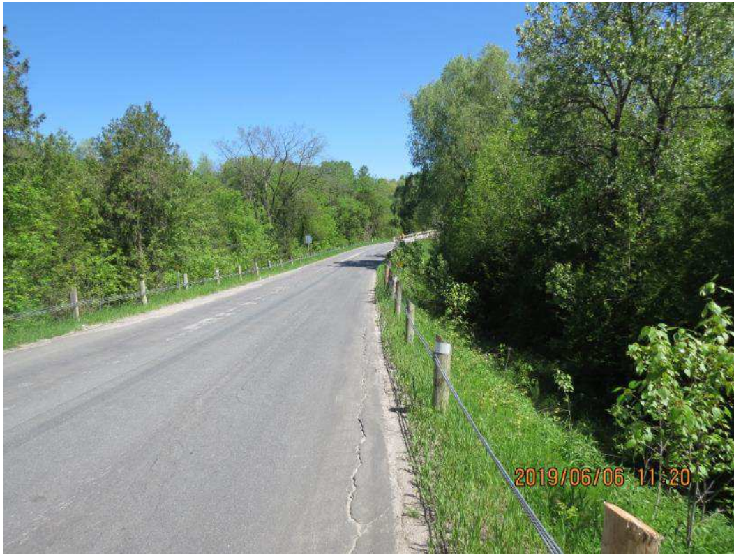
IMG_1603 Road South of Bridge (2 of 3)
