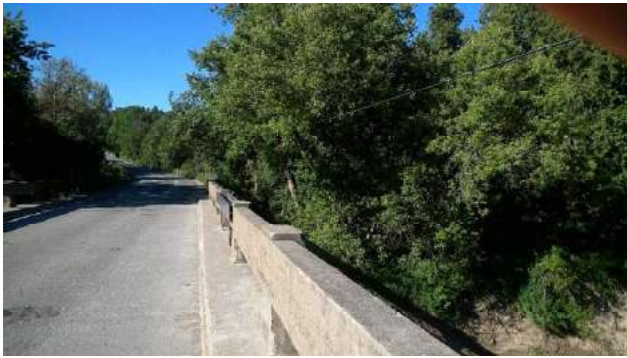
Photo 1. Facing south from center of bridge (June 17, 2021).
