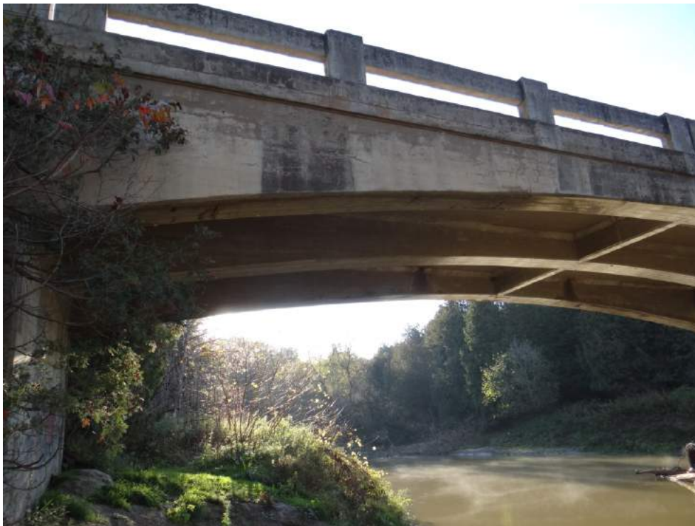
Plate 2: West elevation of the northern span and north abutment, looking east.
