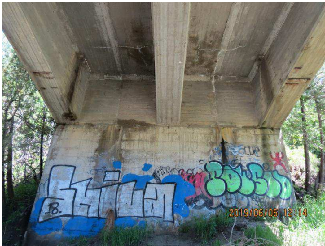
IMG_1820 North End Soffit
