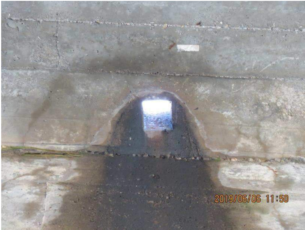
IMG_1702 Typical Deck Drain from Underside of Deck
