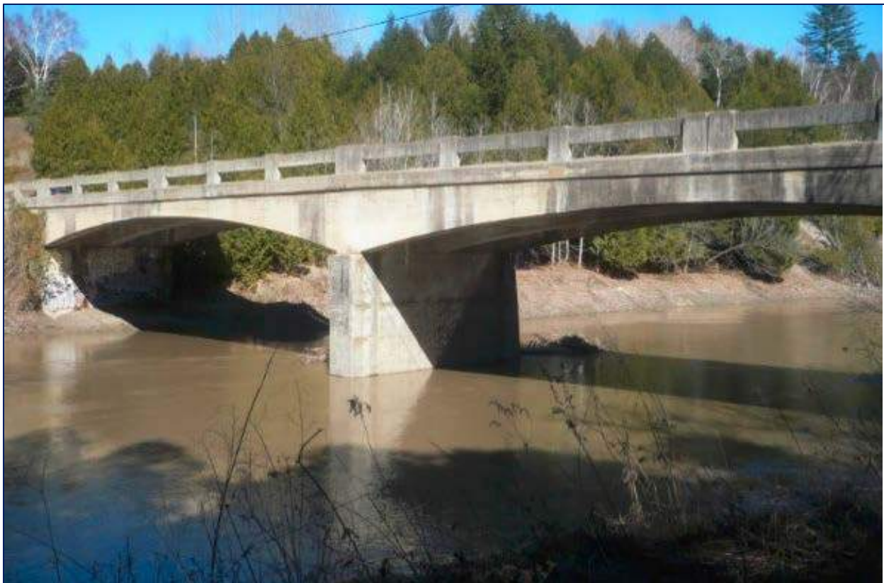
Figure 3: Bridge No. 9 West Elevation View (2019)
