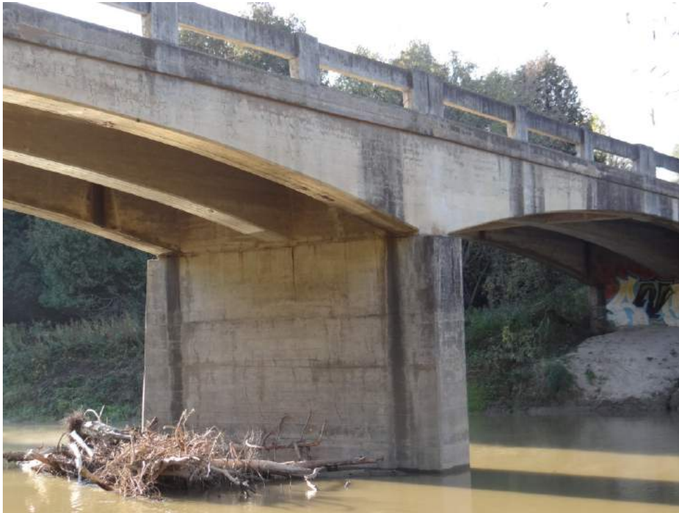
Plate 3: West elevation of the central pier, looking southeast.
