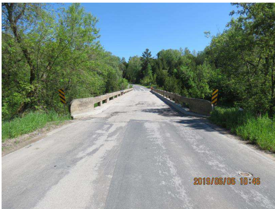
IMG_1413 Road over Structure Looking North
