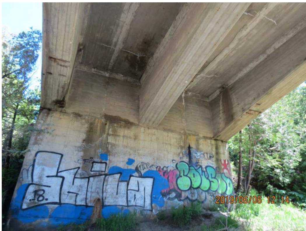
IMG_1816 North Girders (2 of 2)
