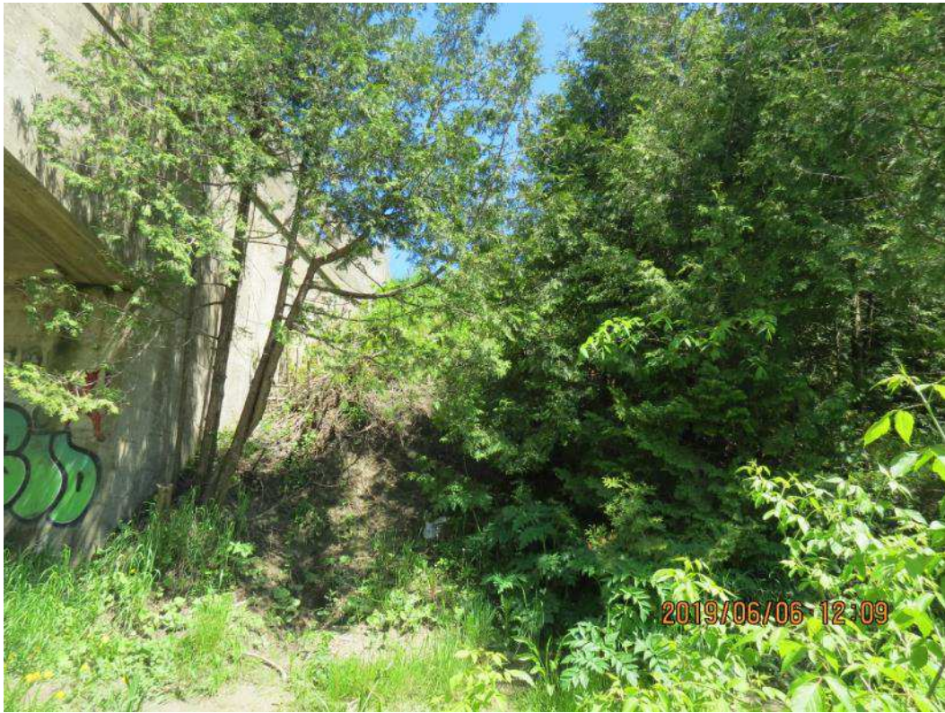
IMG_1777 Northeast Embankment (2 of 2)
