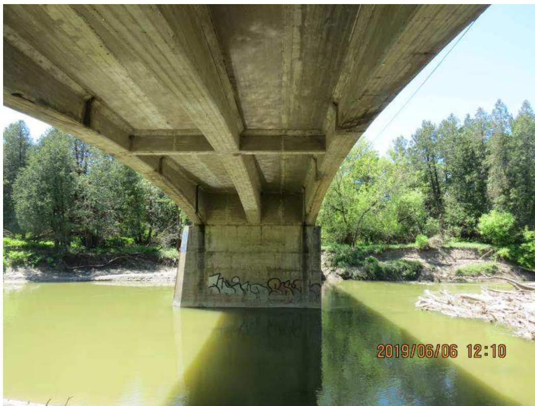
IMG_1789 North Girders (1 of 2)
