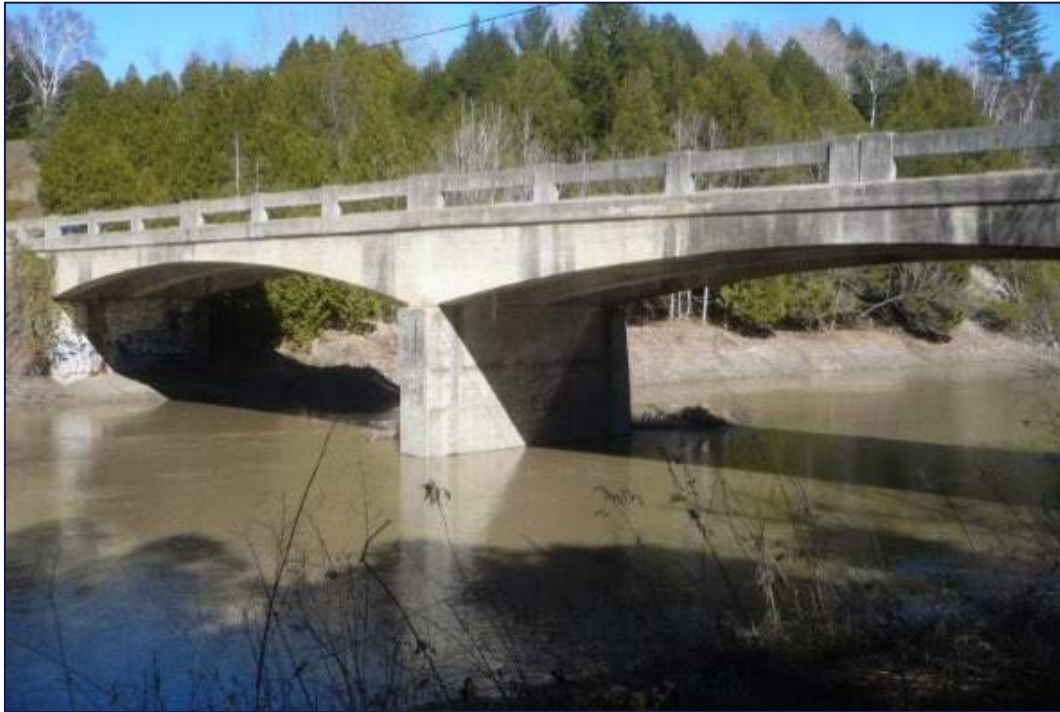
Bridge No. 9 West Elevation View
