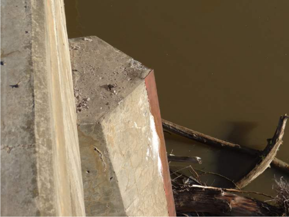
Plate 10: Ice floe protection on the east (upstream) elevation of the pier.
