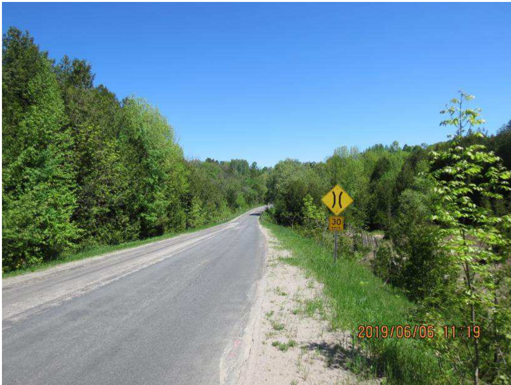
IMG_1597 Road South of Bridge (1 of 3)
