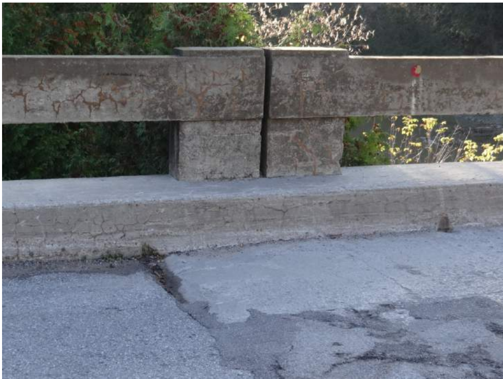
Plate 15: East railing on north portion of the bridge deck, looking east.
