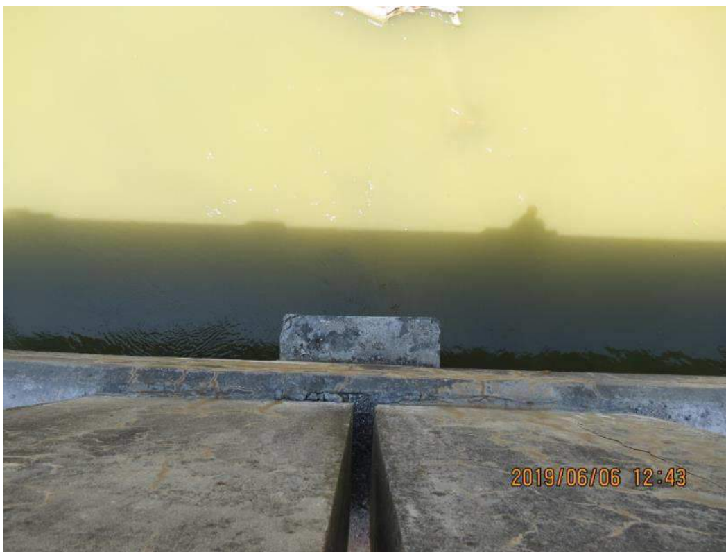
IMG_1862 Center Pier West Side (2 of 2)
