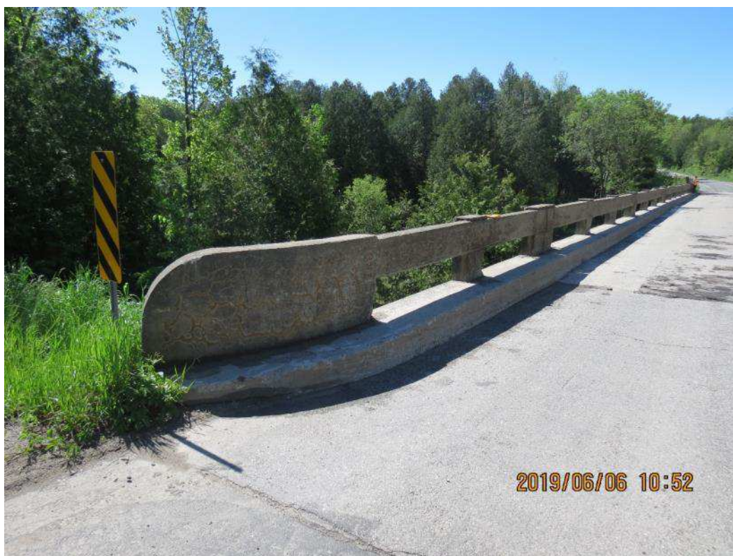
IMG_1458 East Railing North End Panel
