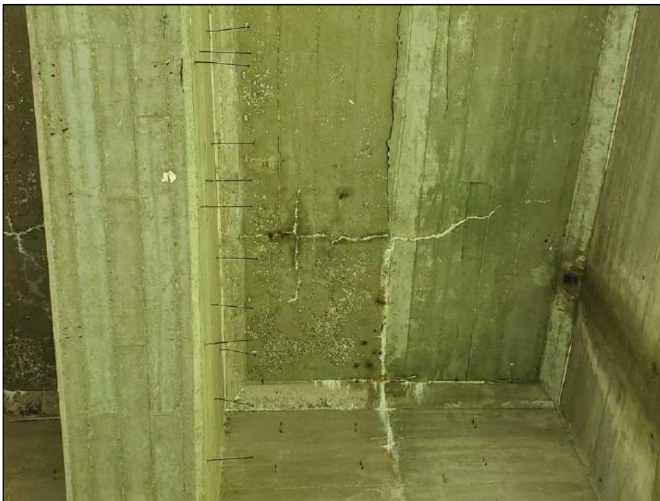
Transverse crack with efflorescence on soffit (typ.)
