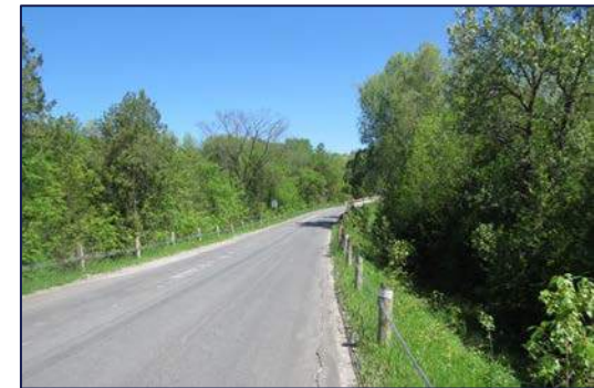
5th Line Approach South of Bridge No. 9 (2019)
