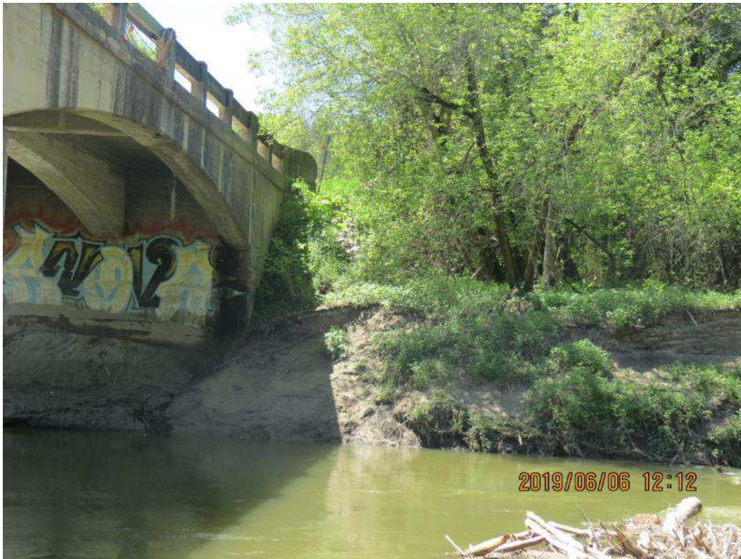
IMG_1803 Southwest Embankment
