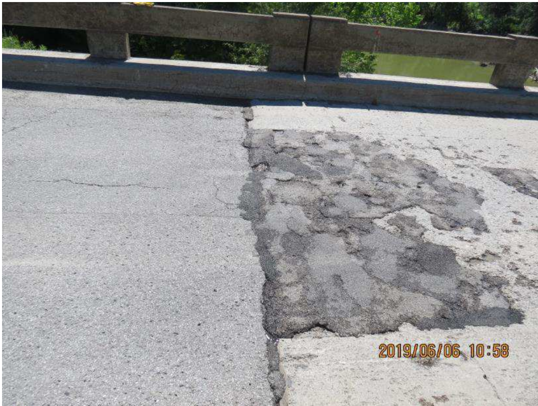
IMG_1508 North Joint at Deck (1 of 2)
