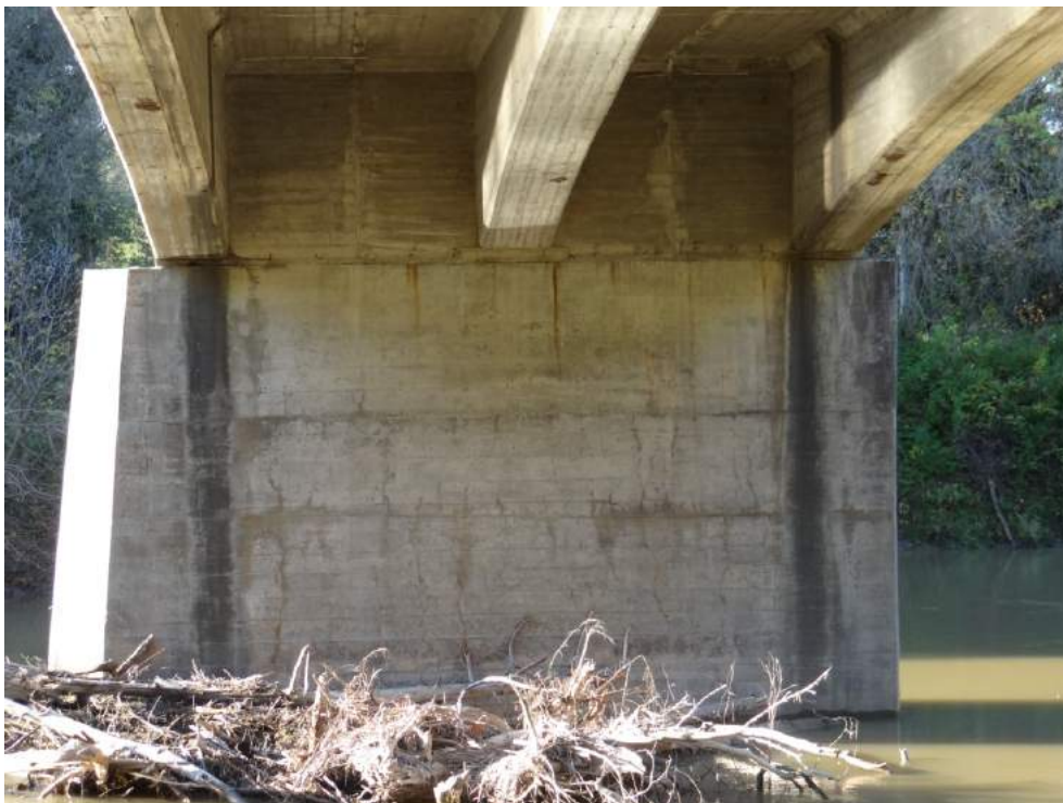
Plate 8: North elevation of the pier, looking south.
