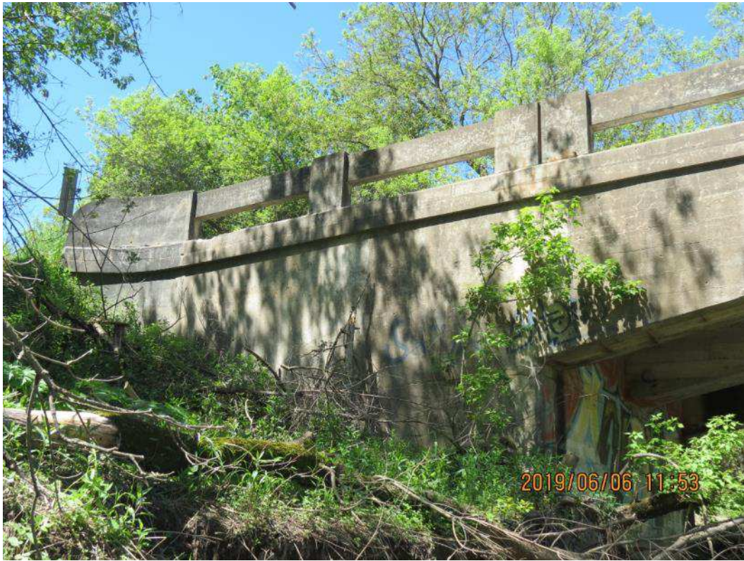
IMG_1725 Southeast Embankment (2 of 2)
