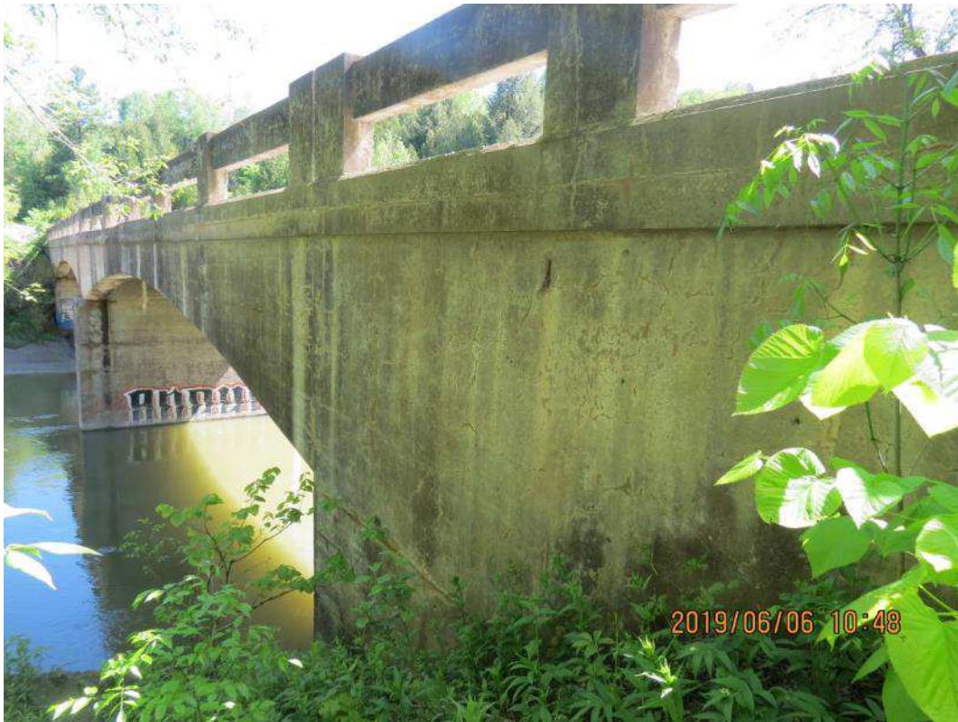
IMG_1423 Southwest Wingwall
