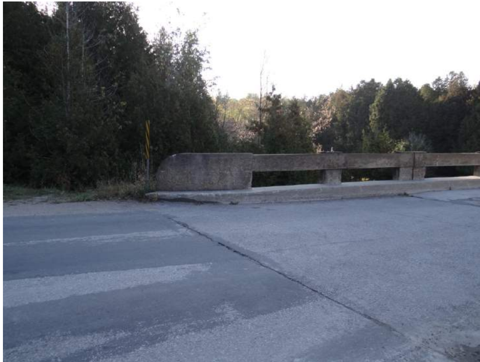
Plate 12: North approach showing eastern railing, looking southeast.
