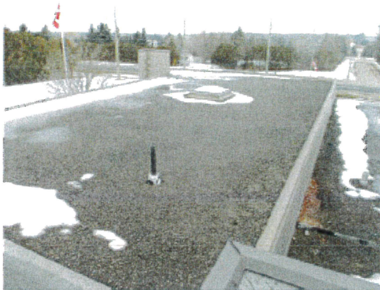
Overview roof area
