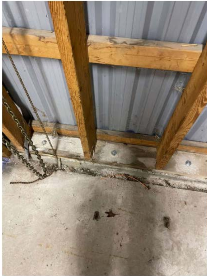
Photograph 3 - Reinstated damaged sill plate
