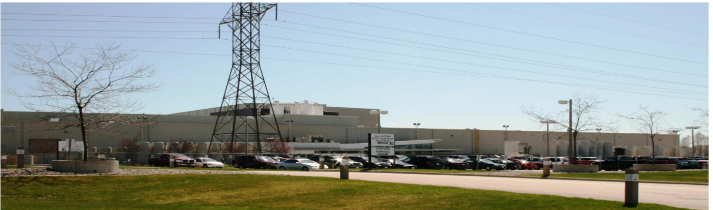
MUNRO Concrete Products Ltd.
