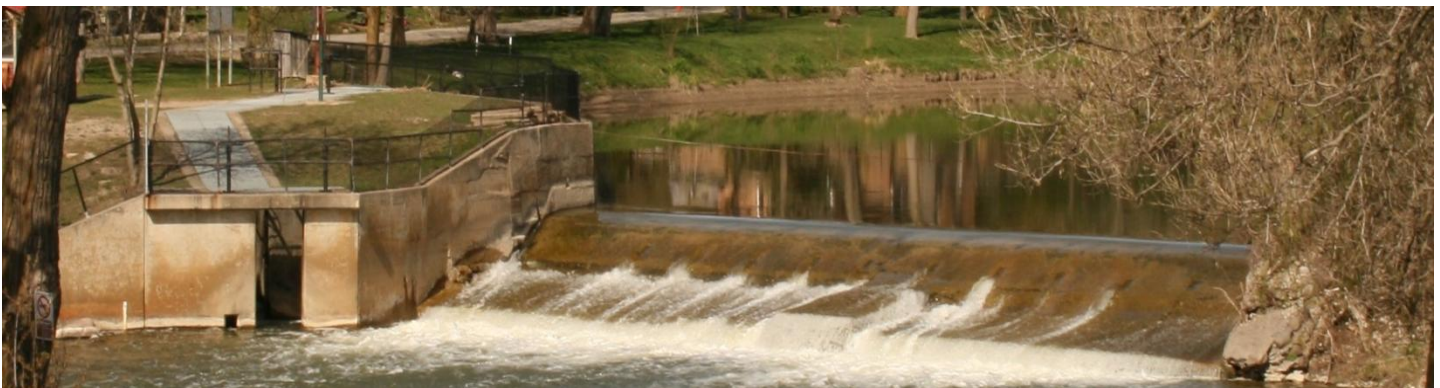
Nicolston Dam on Line 5, Essa
