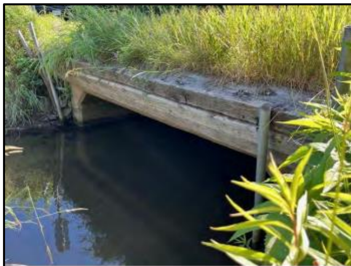
Culvert No. 24 – 8th Line (BCI = 73.2 Good)
