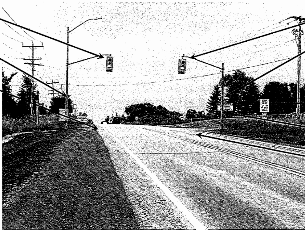
LOOKING SOUTH ON SIDEROAD 20
